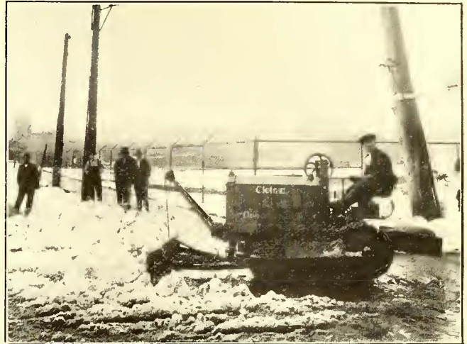
SMALL CATERPILLAR TRACTOR PROVES VERY EFFECTIVE IN CLEANING SNOW FROM DOWNTOWN SPECIAL TRACKWORK
