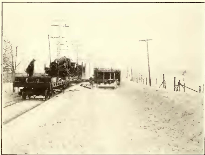
AT LEFT, CLEARING THE HIGHWAY TO KEEP TRAFFIC OFF THE INTERURBAN TRACKS, SHOWING FOLDING WING PLOW IN OPERATING POSITION, FOLLOWED BY HEAVY SPECIAL PLOW PROJECTING OUT INTO THE HIGHWAY. AT RIGHT, FOLDING SIDE WING SNOW PLOW CONTROLLED BY THREE AIR CYLINDERS
