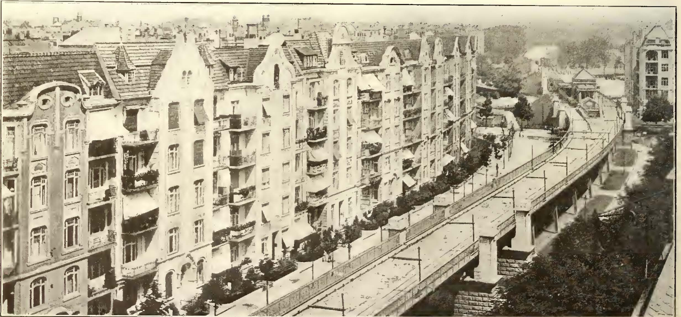
SECTION OF ELEVATED RAILWAY THROUGH RESIDENTIAL SECTION
