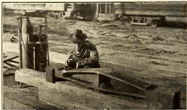
REPAIRING A CRACKED BOLSTER
