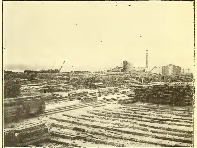
TIES STACKED IN PILES FOR SEASONING
