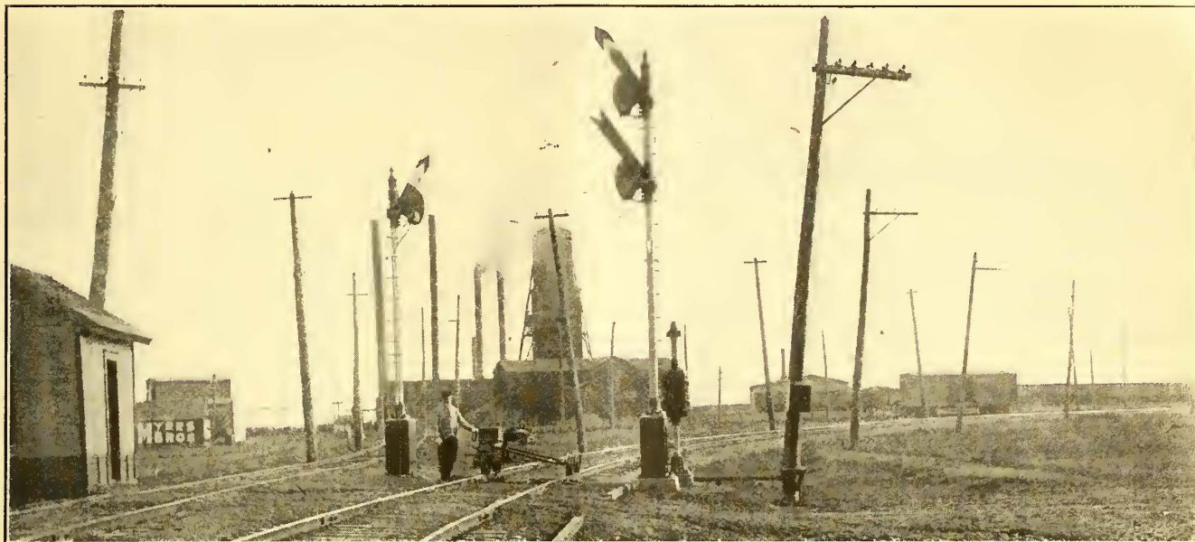
SEMAPHORE SIGNALS AND SIGNAL MAINTAINER AND EQUIPMENT PROVIDED FOR HIM ON THE ILLINOIS TRACTION SYSTEM
