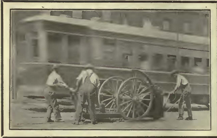
Reciprocating Track Grinder in Action
