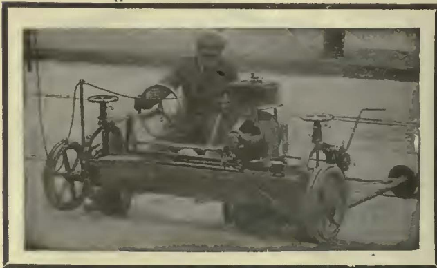
Atlas Rail Grinder on the Job
