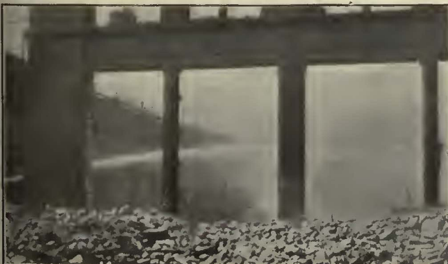
STRUCTURE CAUSED TO SAG BY INTENSE HEAT
