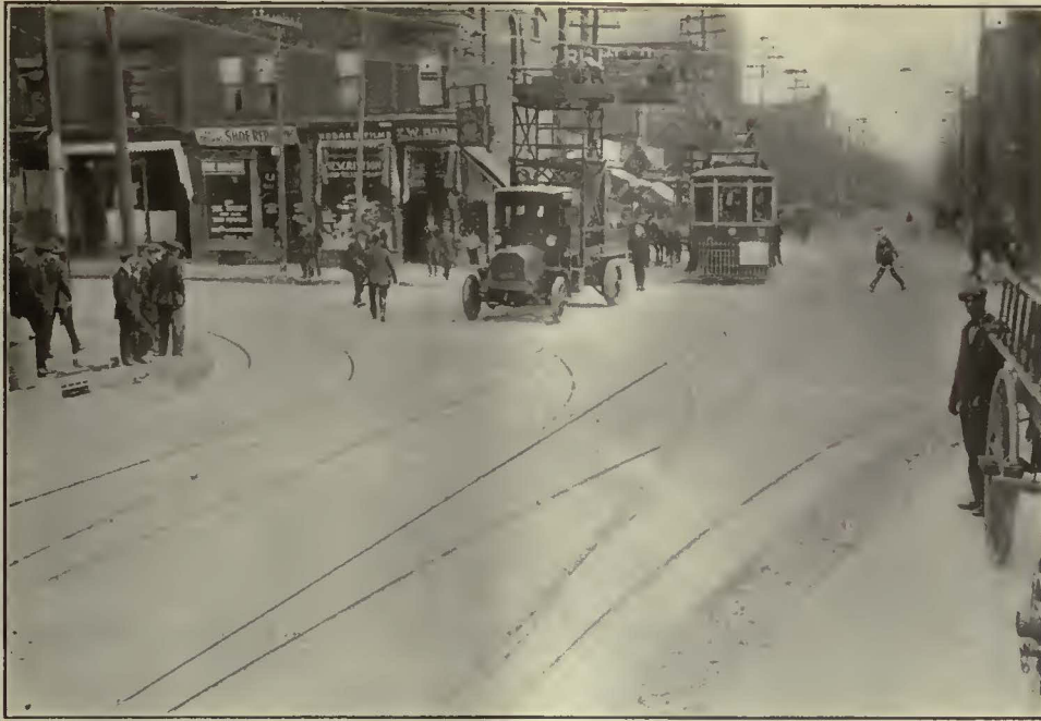
TYPICAL FINISHED TRACK CONSTRUCTION IN TORONTO—INTERSECTION AT QUEEN AND CHURCH STREETS
