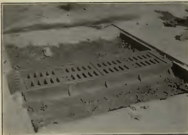
TRACK DRAIN IN POSITION READY FOR PAVING
