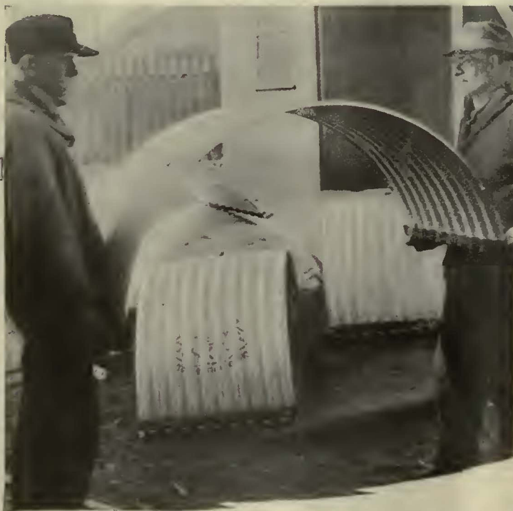
Two men easily handle 48-inch diameter "ACME" (Nestable) Culvert
