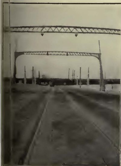
FINISHED TRACK CONSTRUCTION, SHOWING ASPHALT STRIP ALONG THE RAILS
