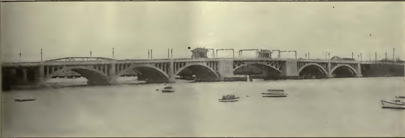
THE OVERHEAD WIRE AND TRACK CONSTRUCTION ON THIS NEW BRIDGE ACROSS THE HOUSATONIC RIVER HAS JUST BEEN COMPLETED BY THE CONNECTICUT COMPANY
