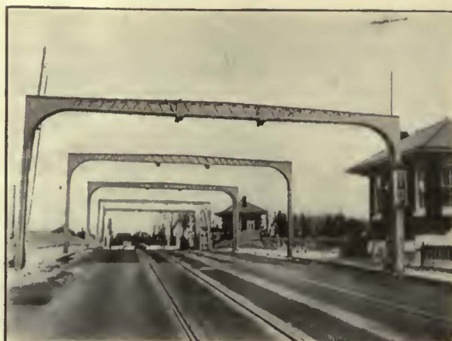
THE ENTRANCE TO LIFT CLOSED AND TRACKS OPEN FOR OPERATION
