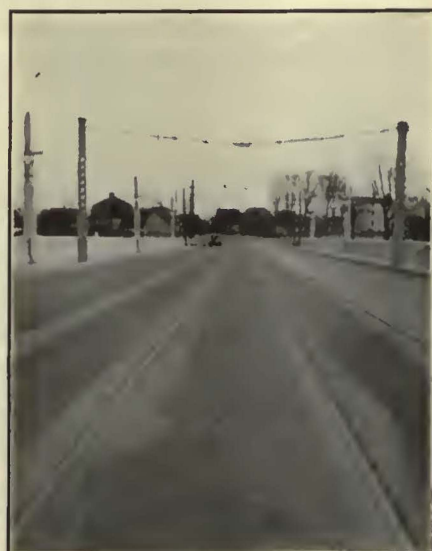
FINISHED TRACK CONSTRUCTION, SHOWING ASPHALT STRIP ALONG THE RAILS
