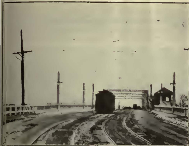
APPROACH TO BRIDGE WITH TRACK AND OVERHEAD IN COMPLETED CONDITION
