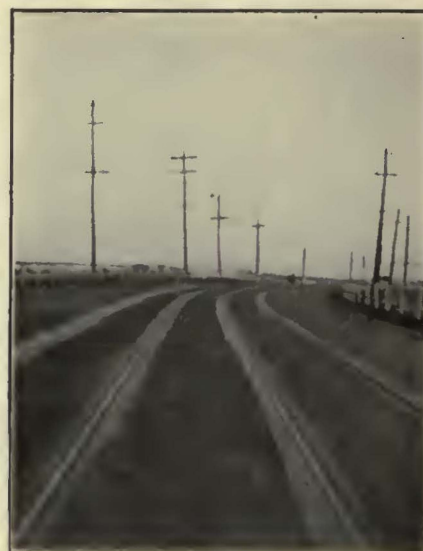
FINISHED TRACK CONSTRUCTION, SHOWING ASPHALT STRIP ALONG THE RAILS
