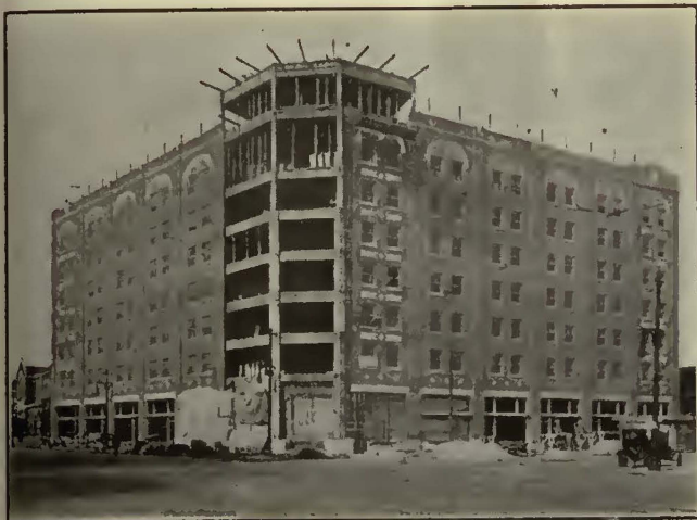
NEW HOTEL ADJACENT TO INTERURBAN TERMINAL NEARING COMPLETION
