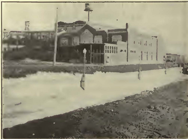
RETAINING WALL ALONG ARKANSAS RIVER WHICH PROTECTS NEW STATION—NEW HOTEL IN BACKGROUND
