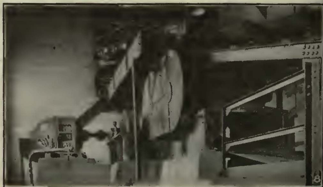
No. 5. Feeder group oil switches with structure and mechanism as the floor level, easy to get at.
