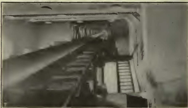
No. 1. Two 20,000-kw. turbo-generators were the initial installation in Lakeside plant.
