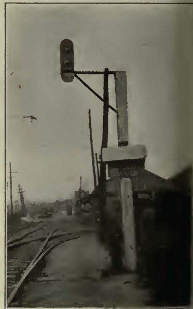
SAFETY SWITCH STAND AT SHOP YARD TURNOUT EQUIPPED WITH MAIN LINE ELECTRIC SIGNAL INTERLOCK
