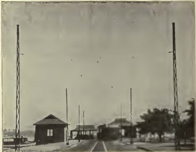
Bates Poles in Trolley Construction, Sydney, N. S. W.
