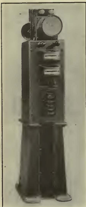
SIGNALING AND SYNCHRONIZING PANEL FOR EACH MAIN GENERATOR
