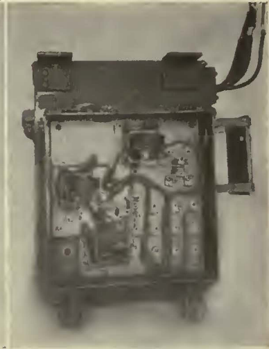
NOTCHING AND OPERATING RELAYS OF LINE SWITCH
