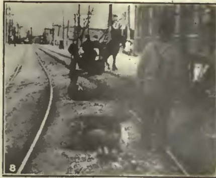
No. 7—This one will not disturb the track. No. 8—An operation which will require careful back-filling. No. 9—Close work in this devil strip.
