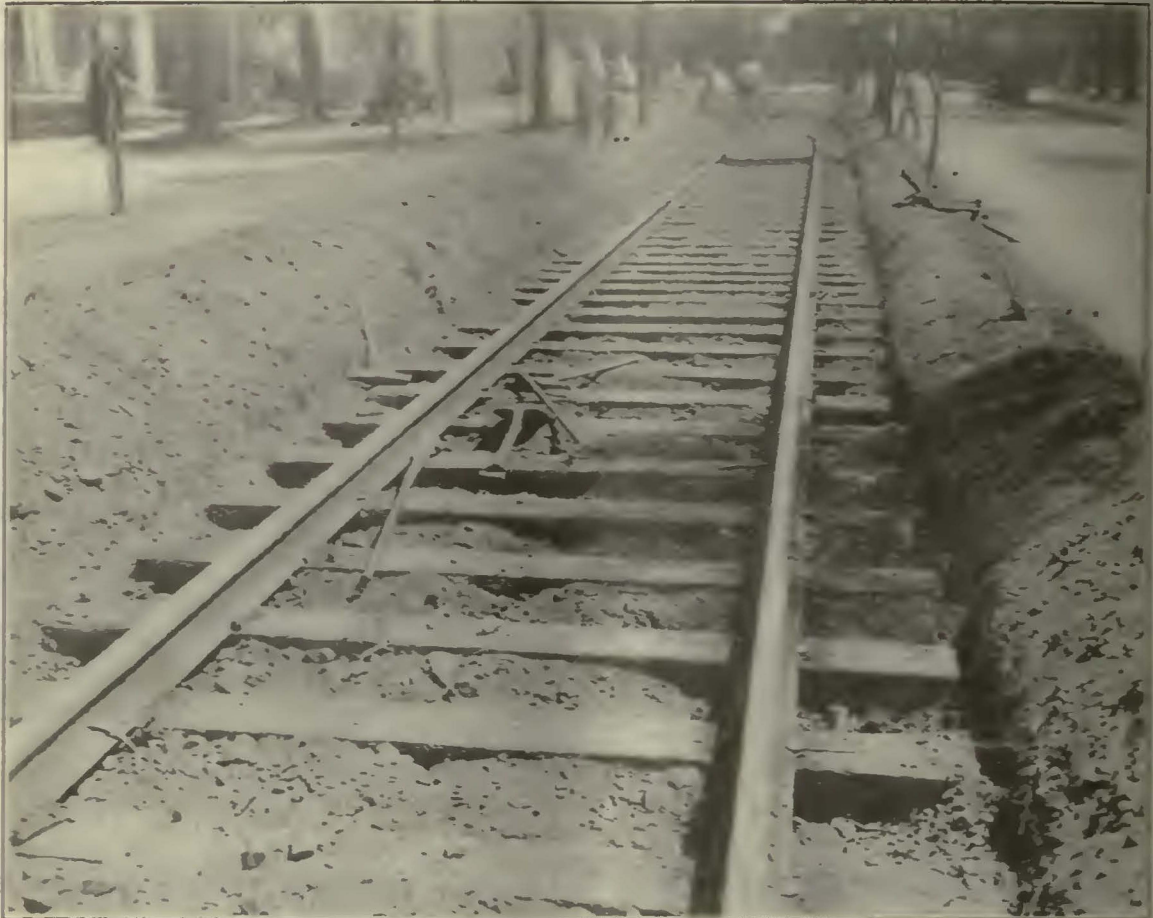
(Recent photograph showing creosoted pine ties supplied by this company in track, New Orleans Street Ry. since 1899)
