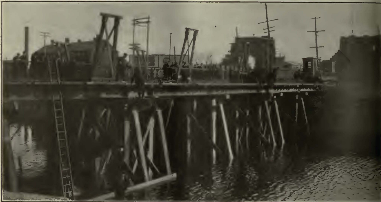
BUILDING A BRIDGE IN ELEVEN HOURS AT HOLYOKE, MASS.
