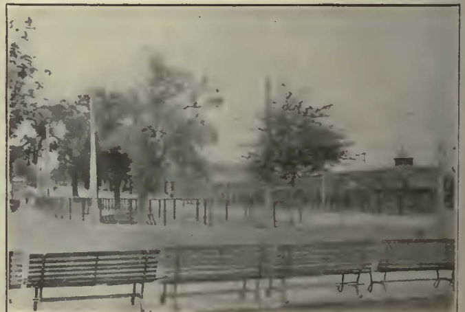
GENERAL VIEW OF THE TERMINAL AS SEEN FROM THE PARK SIDE
