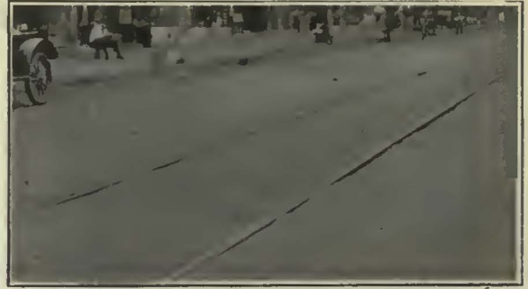
FIG. 2—CROSSING ON GERMANTOWN AVENUE WITH WOOD BLOCK PAVEMENT, LAID IN 1916
