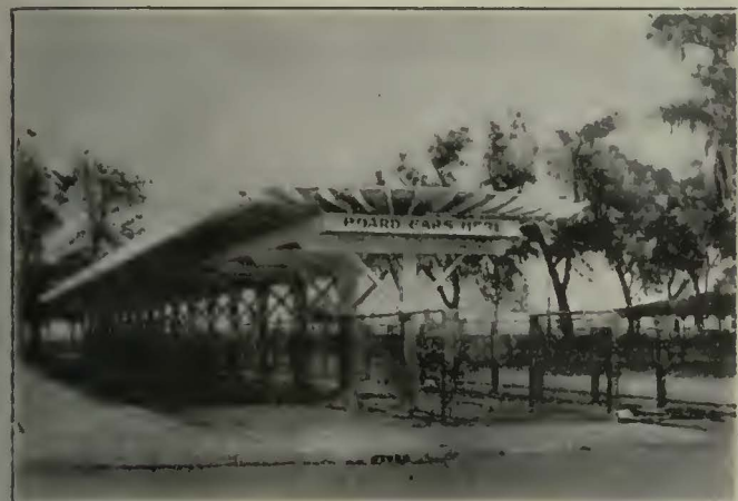
LOADING PLATFORM, SHOWING SHELTER, TURNSTILE STATION AND CHANCE BOOTH
