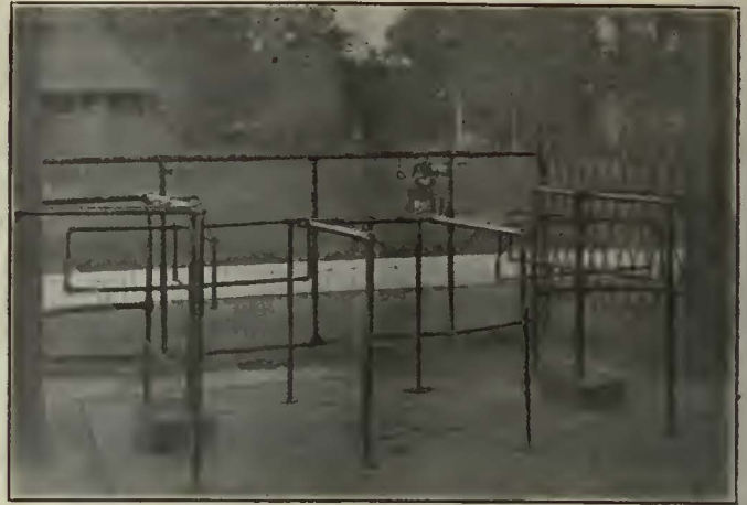
CLOSE-UP VIEW OF FARE COLLECTOR'S STATION, SHOWING TURNSTILES, AUXILIARY FENCE AND ONE PANTOGRAPH GATE
