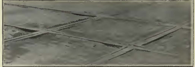
FIG. 4—CROSSING COMPLETED IN 1921
