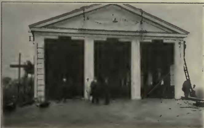
CONCRETE CARHOUSE AT GREEN RIDGE
