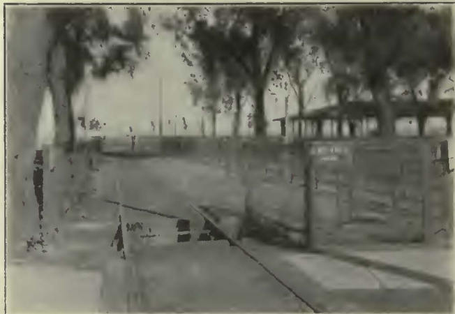
GENERAL VIEW OF UNLOADING PLATFORM, SHOWING WATER BARRIER AND TURNSTILE
