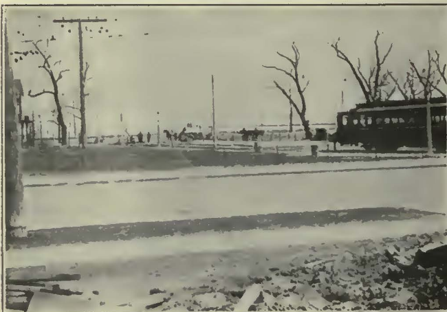
SITE OF THE NEW CHARLOTTE TERMINAL BEFORE THE BEGINNING OF CONSTRUCTION
