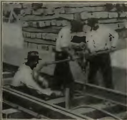
Other machines such as the screw spike driver can be used with a Tamper Car to reduce track work costs.
