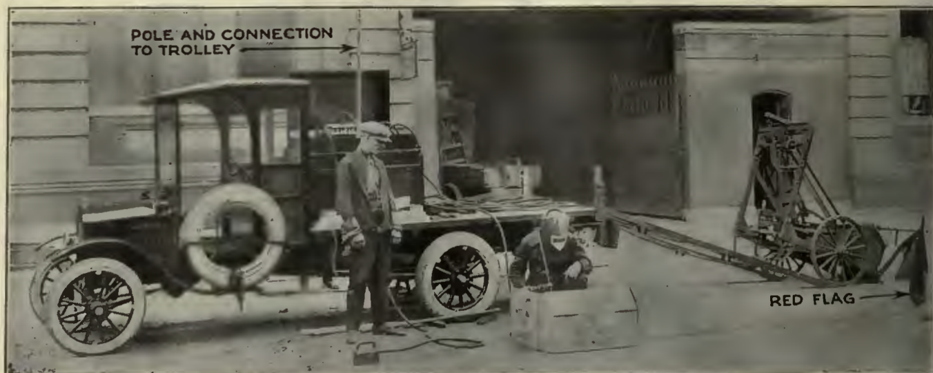
THE B. R. T. WELDING AND GRINDING APPARATUS READY FOR WELDING
