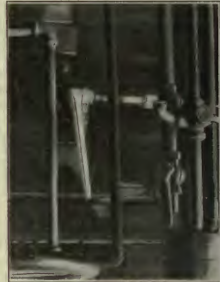
MECHANISM FOR TILTING ARC HEADLIGHTS ON INTERURBAN CARS, AND, AT RIGHT, LEVER AND CONNECTING MECHANISM FOR TILTING HEADLIGHTS
