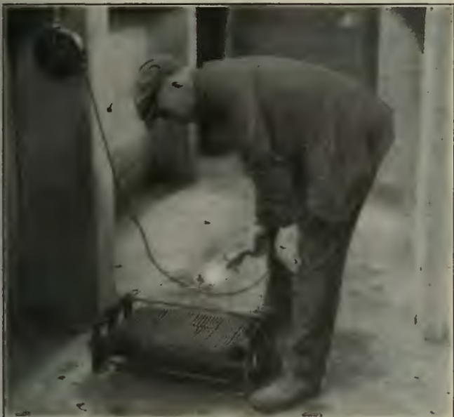
INSPECTING RESISTANCE GRIDS WITH PORTABLE LIGHT WITH CORD EXTENSION FROM REEL
