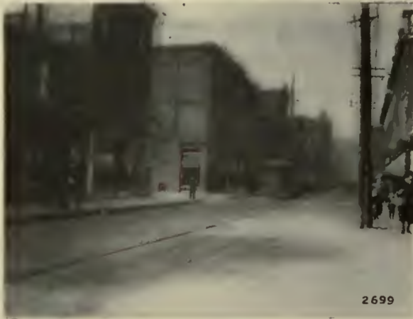
Carson Street, Pittsburgh, where Thermit Insert Welds have recently been installed. This city has many miles of Thermit track, some sections having welds ten years old and still in excellent condition.
