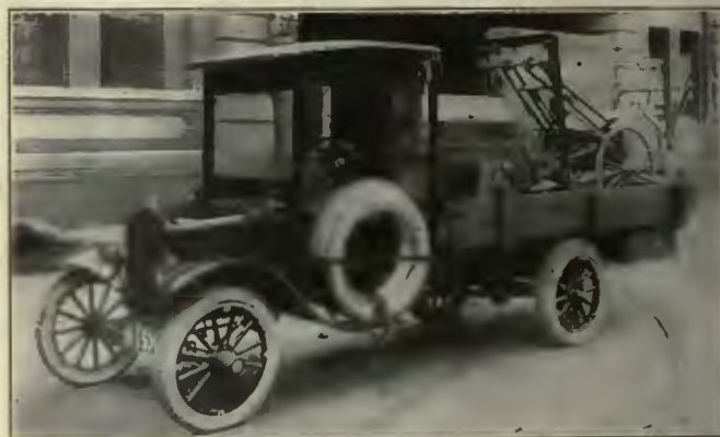
B. R. T. EMERGENCY WELDING AND GRINDING OUTFIT READY TO MOVE
