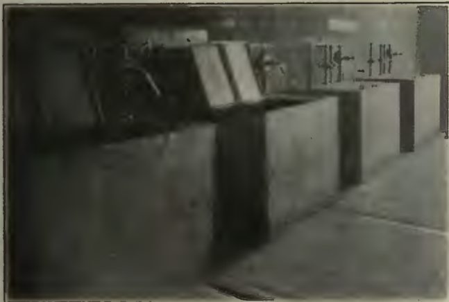
WASTE SATURATING TANKS WITH PUMPING EQUIPMENT AND CONTROLS TO THE VARIOUS COMPARTMENTS OF EACH TANK
