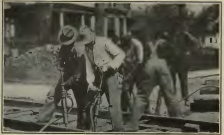
Imperial Tamperers enable small gangs to equal the work output of large ones.
