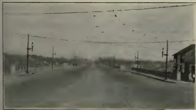
NEW VIADUCT WHICH HAS BEEN BUILT OVER THE CUYAHOGA VALLEY, AKRON, OHIO
