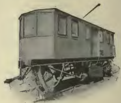
End view of Standard Single Truck Sweeper.
