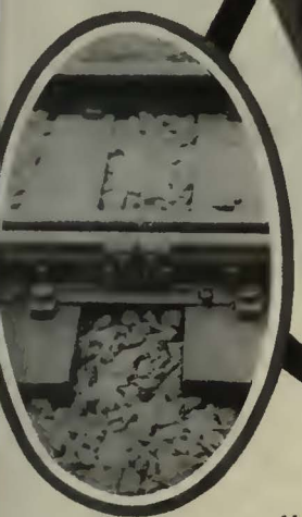
Below—O-B Gas Weld Bond on Running Rail
