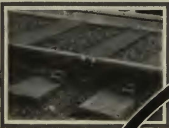
Above right—O-B Signal Bond on Running Rail
