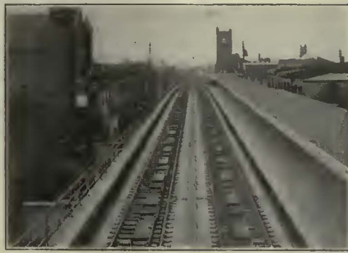
A PORTION OF THE TRACK IS CONSTRUCTED WITH SHORT TIE BLOCKS SET IN CONCRETE, BUT NOT BOLTED THERETO
