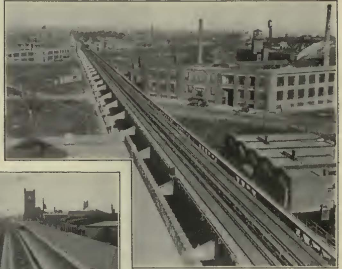
THE CHAMFERED ENDS OF THE TRANSVERSE GIRDERS GIVE THE SUPERSTRUCTURE A FINISHED APPEARANCE
