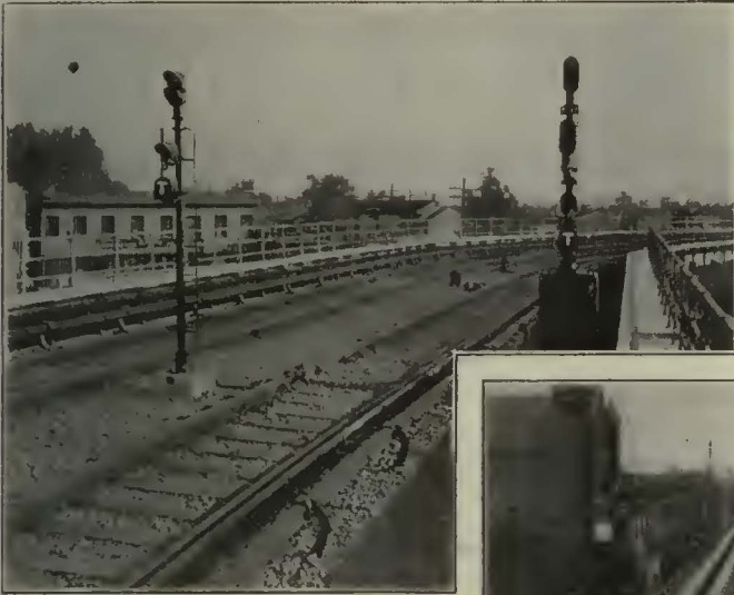
THIS ROCK-BALLASTED TRACK ON THE FRANKFORD ELEVATED RAILWAY GIVES ONE AN IMPRESSION OF PERMANENCE
