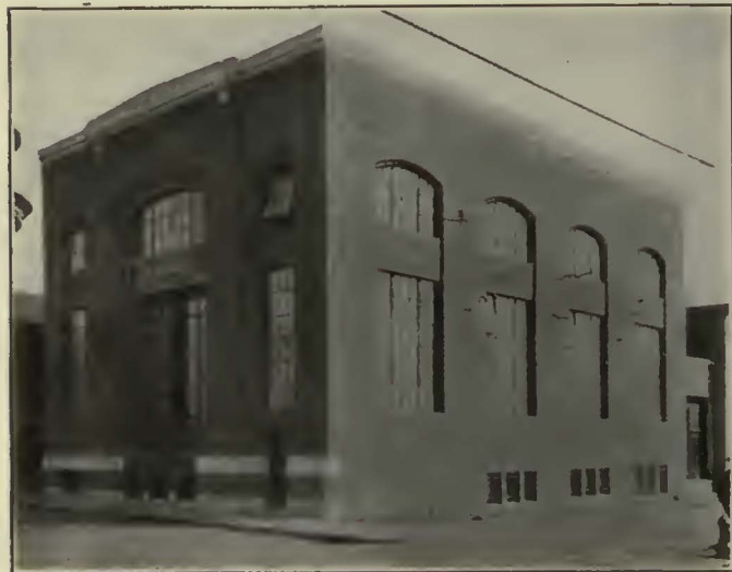
SUBSTATION ARCHITECTURE IS SIMPLE BUT DIGNIFIED
