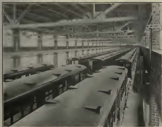
THE INSPECTION SHOP IS CAPACIOUS AND WELL LIGHTED
