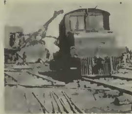
On Electric Locomotives
