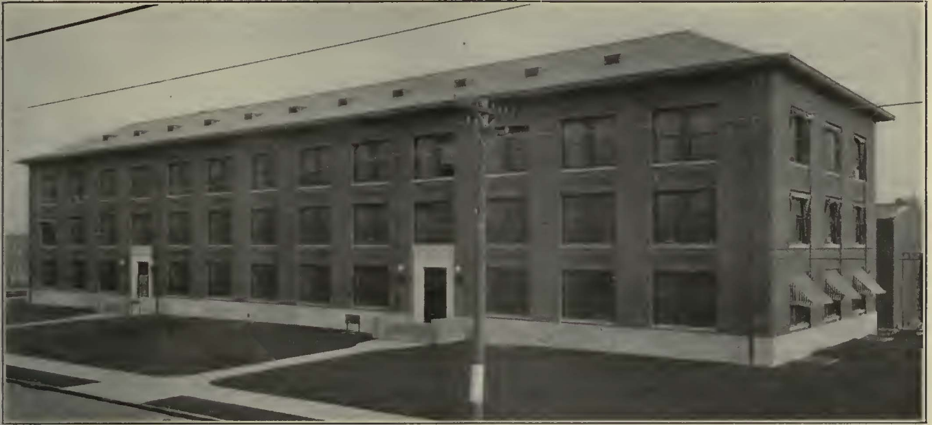
NEW GENERAL OFFICE BUILDING WHICH HOUSES ALL DEPARTMENTS OF DETROIT MUNICIPAL RAILWAY
