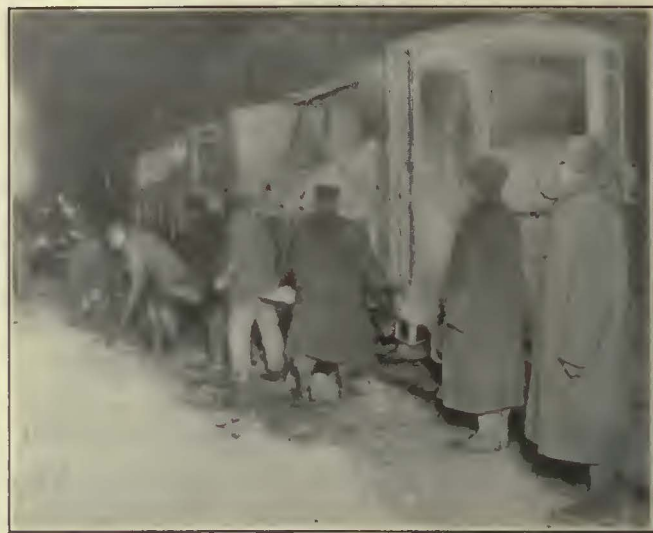
DUMPING SLEDS AND DUMPING CARS FOR HAULING SNOW IN BOSTON
