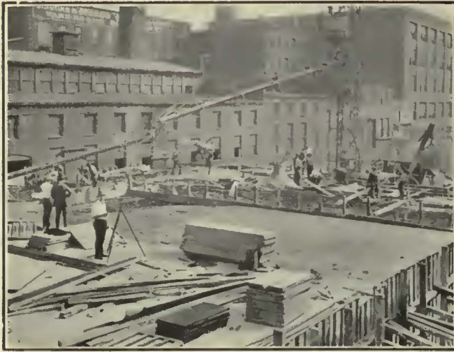
CONSTRUCTING STREET OVER SUBWAY—VIEW FROM ABOVE
