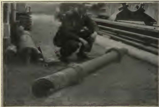
SHAFT BROKEN OUTSIDE OF PREVIOUS WELD
