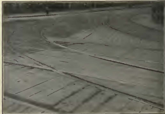
DOUBLE-TRACK BRANCH-OFF CONSTRUCTED WITHIN WEEK IN ROCHESTER, N. Y.
