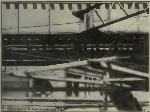
PROTECTIVE COVERINGS FOR OVERHEAD WORK No. 1. Wooden sheathing under girder. No. 2. Long trough construction. No. 3. Putting up long troughs in place of flashboards. No. 4. Flashboard construction. No. 5. Short troughs.
