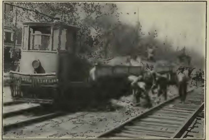
PICKING UP A LOAD WHILE TRACKS ARE BEING RECONSTRUCTED
