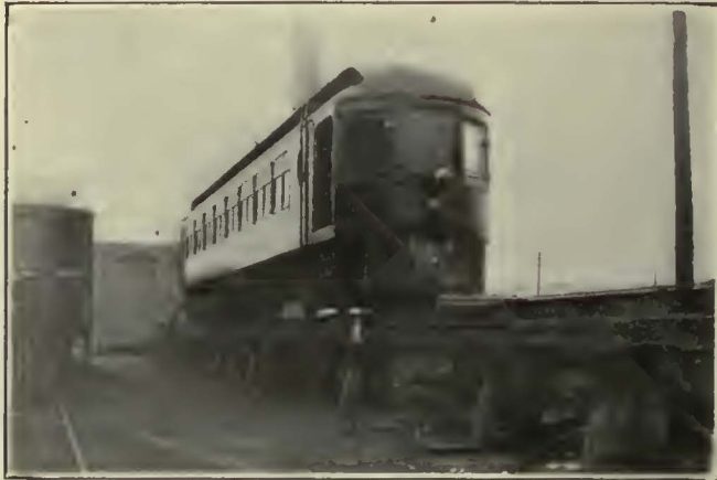
ELEVATED YARD TRACK FOR UNDERBODY CAR REPAIRS
