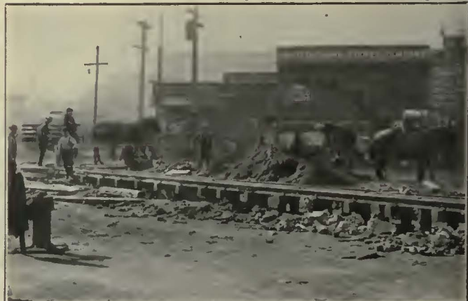
RECONSTRUCTED CABLE TRACK READY FOR CONCRETE
