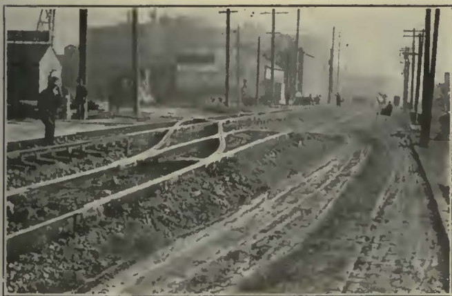
TYPICAL TRACK RAISING OPERATION ON DOUBLE-TRACK LINE
