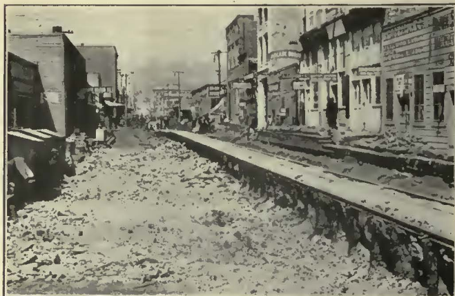
RECONSTRUCTION OF CABLE TRACK IN SERVICE
