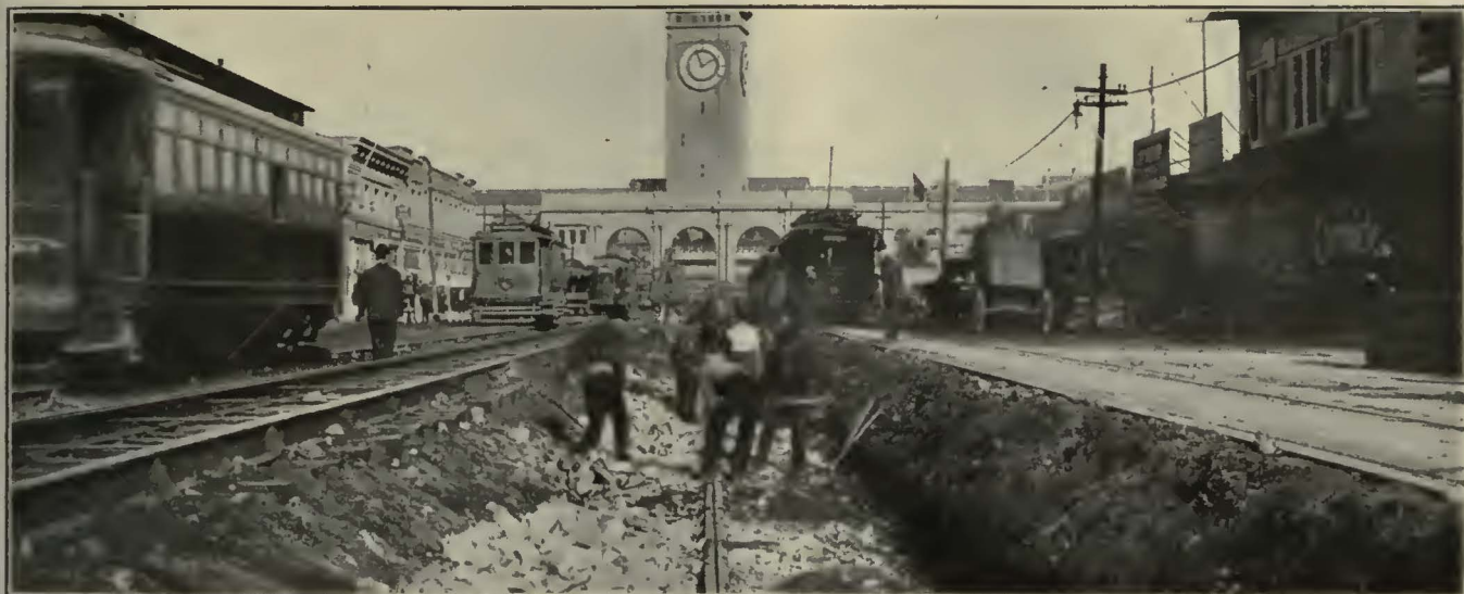
RAISING LOWER MARKET STREET TRACKS AFTER THE FIRE
