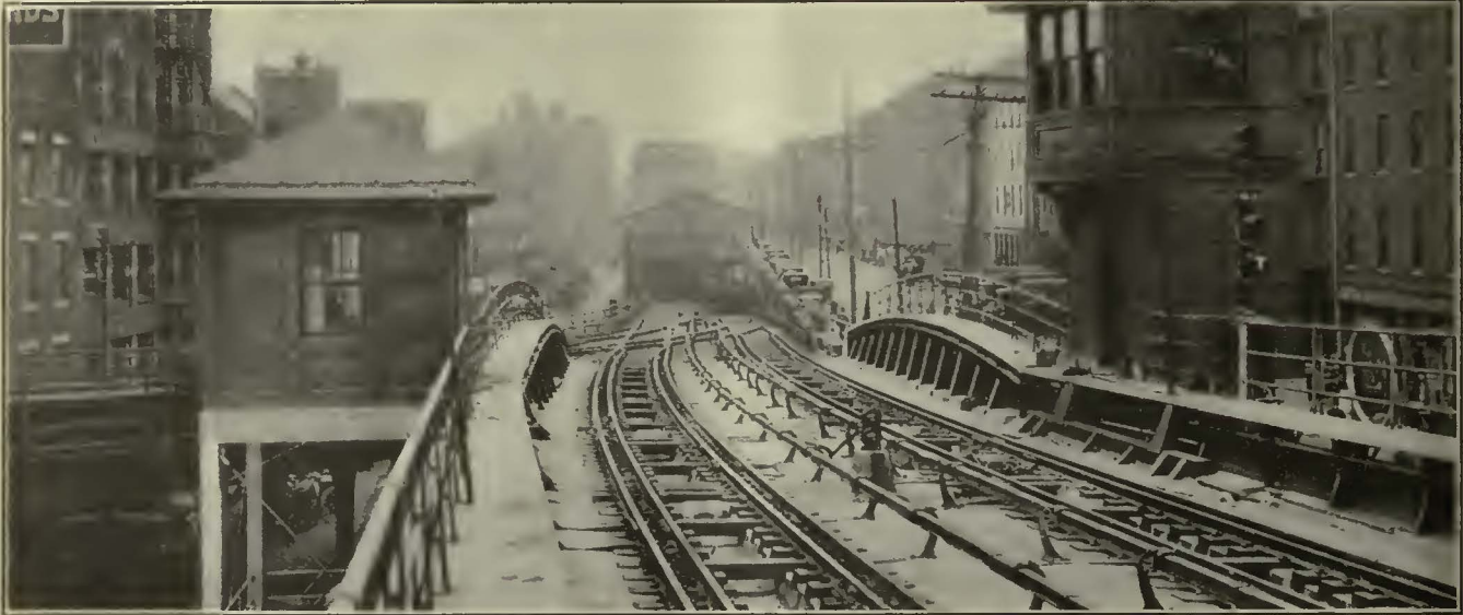
High and Dwarf Color-Light Signals and Automatic Train Stops at Entrance to Market Street Subway, Junction of P. R. T. and Frankford Lines
