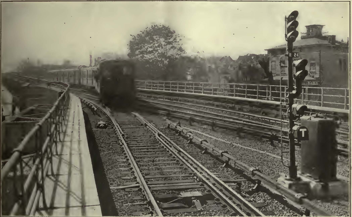
Automatic Train Stop, Color Light Signals, and Switch and Lock Movement, Electro-Pneumatic Interlocking, on Frankford Elevated
