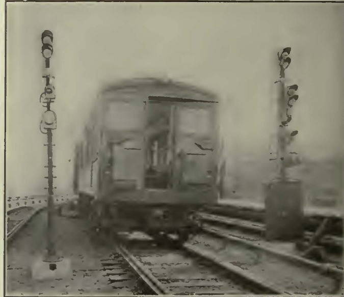
Another Installation of Color-Light Signal at Interlocking on the Frankford Elevated
