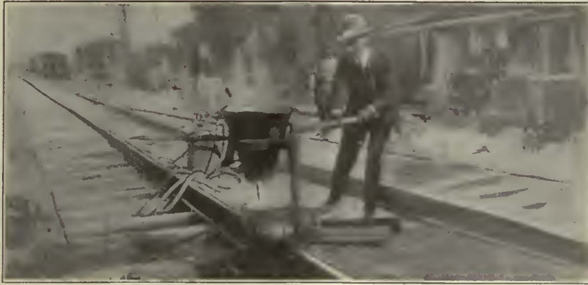
Making a Thermochemical weld in Indianapolis—The Thermochemical reaction
