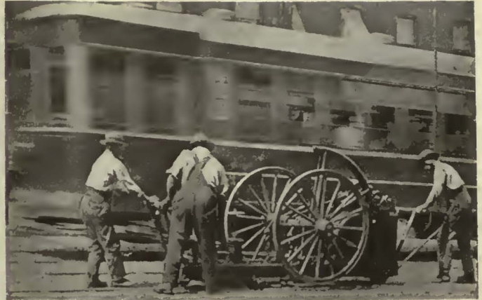
For removing all trace of corrugations from straight and curved track it has no equal. Most economical because the grinding blocks adapt themselves to the shape of the original rail head, and avoid unnecessary grinding and waste of metal.
