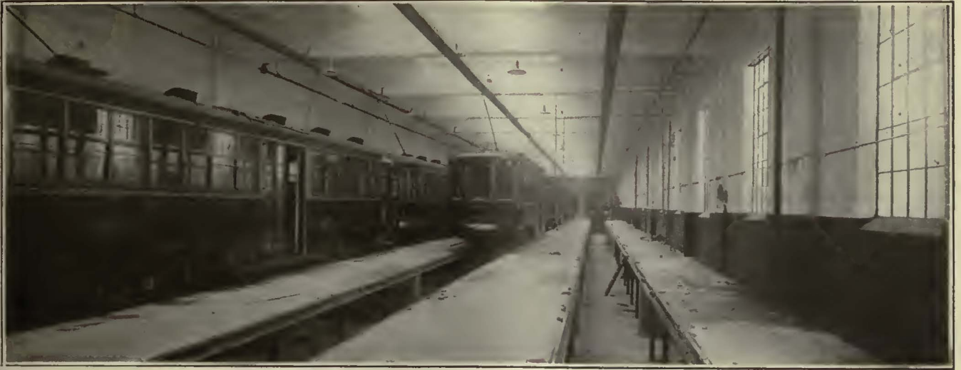
Inspection Bay No. 2 In Carhouse Just Constructed at Toronto
