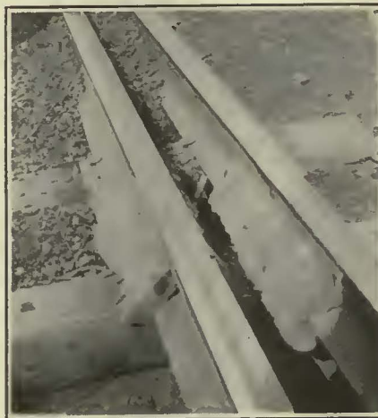
Compromise Joints Made by Pouring Molten Steel About Rails
