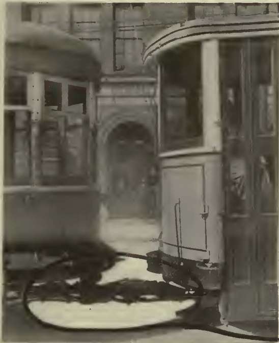
Illustrated: A pair of Westinghouse C-3-A Type Automatic "Tight-Lock" Car and Air Couplers, still giving satisfactory service after nine years on cars of Cincinnati Traction Company.
