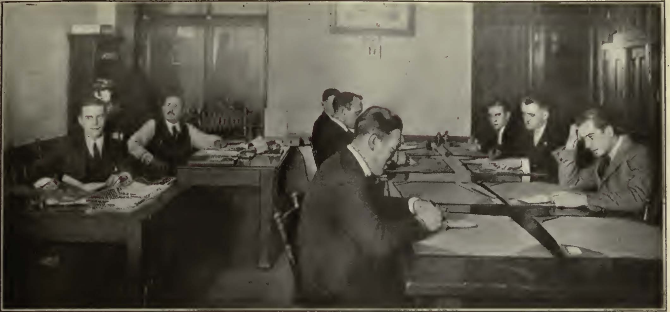
Office Facilities for the Checkers, Inspectors and Timekeepers
