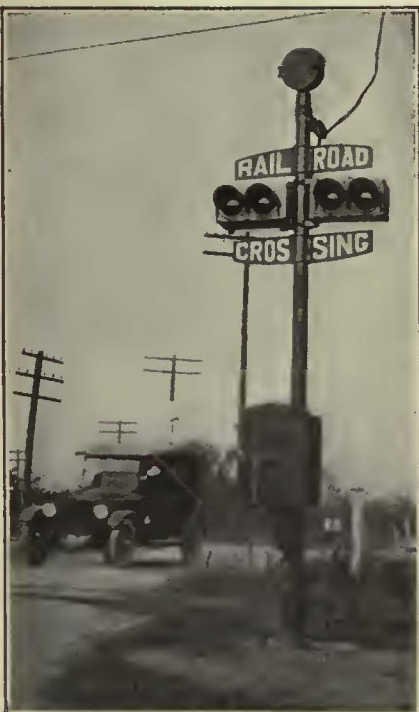
One of the 13 Nachod Crossing Signals on the line of the Interstate Public Service Company, Indianapolis, Indiana.
