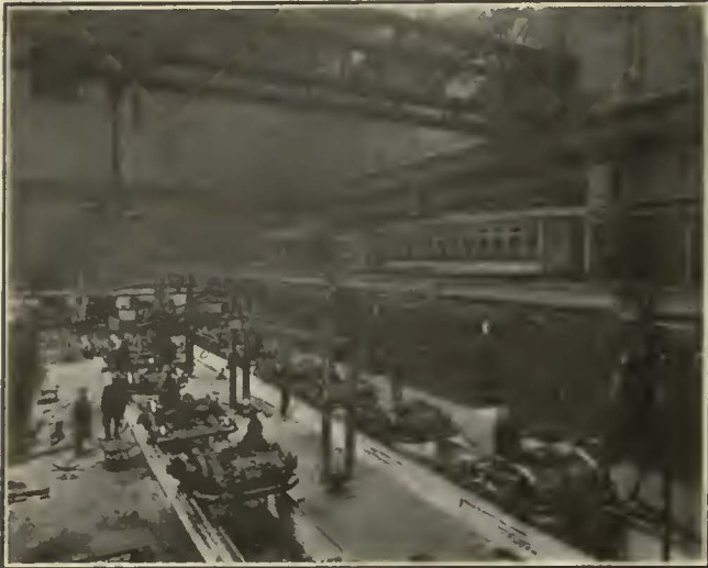
The Truck-Overhauling Tracks of the Third Avenue Railway, New York, Are Raised to a Convenient Height for Efficient Truck Overhauling
