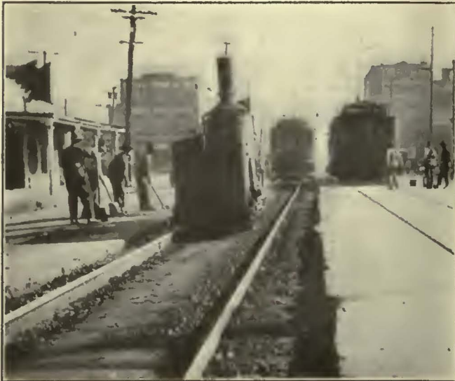
Placing and Rolling, Under Service, the Asphalt Concrete Type of Base
