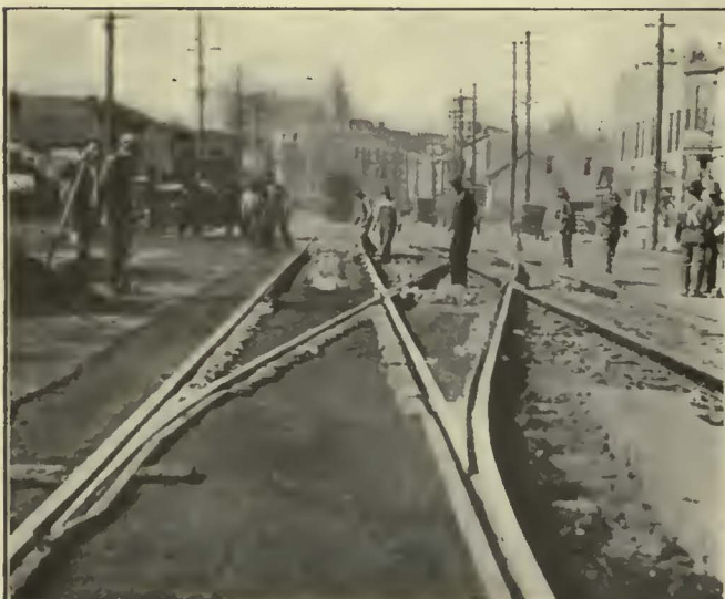
Placing Asphalt Concrete Type of Base Around Special Work
