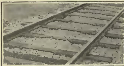
Old Rails with Wooden Side Pieces Used in Tie Construction
