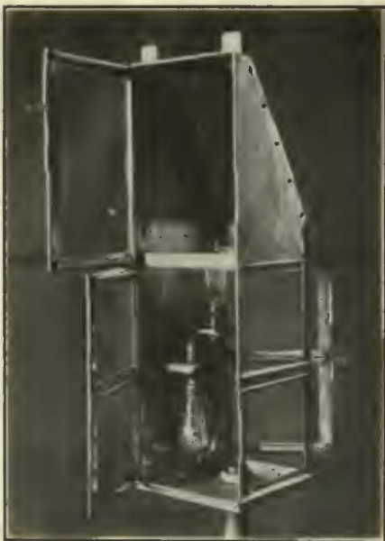
Box Open, Showing Position of Lights and Diagonal Mounting of Mirror
