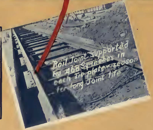
Standard Steel Tie Construction Steel Twin Ties in 7'0" Trench
