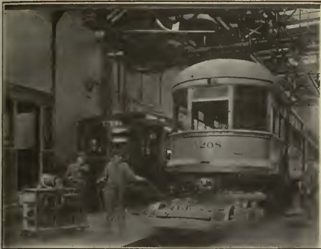
Removing Truck from Underneath Car Body with the Aid of a Portable Control Outfit in the Cleveland Railway Shops
