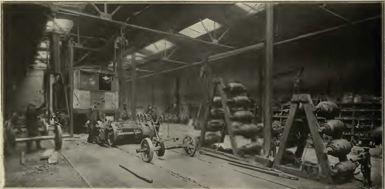
Air Hoists Are Used to Lift Car Bodies in the Federal Street Shops of the New York State Railways, Rochester, N. Y.
