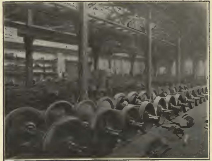
The Truck-Overhauling Tracks of the Long Island Railroad Are Served by an Overhead Traveling Crane
