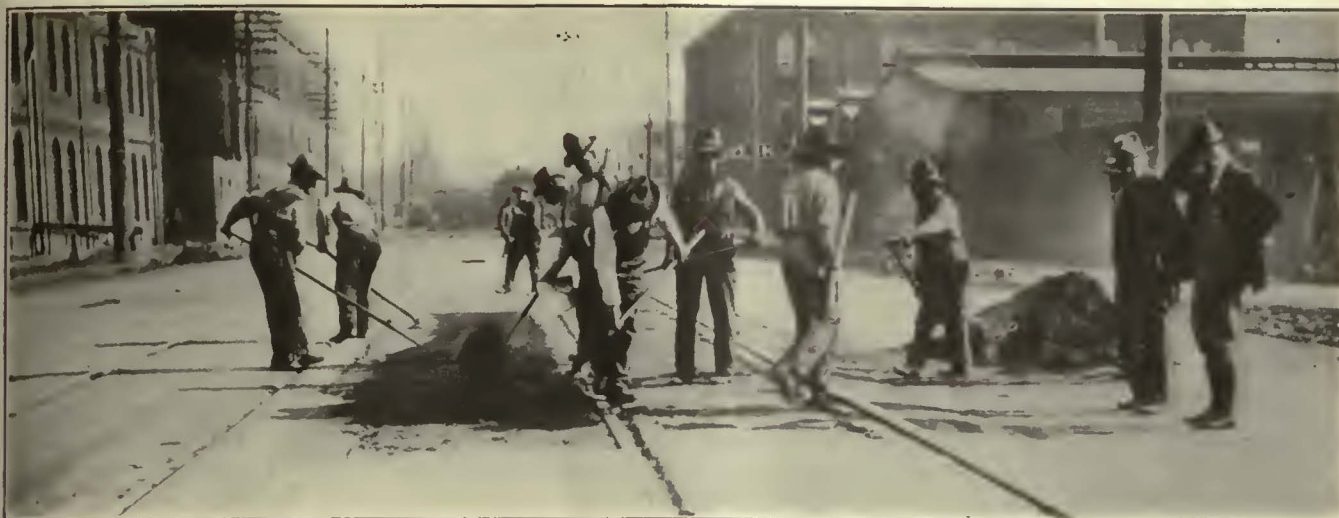
The Asphalt Wearing Surface Being Placed Upon Completed Asphalt Concrete Base
