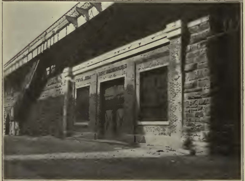
This Substation Is Tucked Away Under the Park Avenue Elevated Structure
