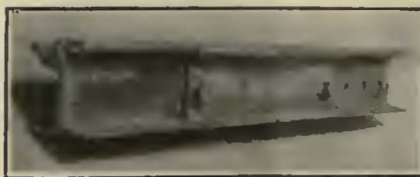
Completed Welded Joints as Installed by Lehigh Valley Transit Company
