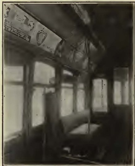
The Grease Reservoir and Piping Are Installed Inside Car
