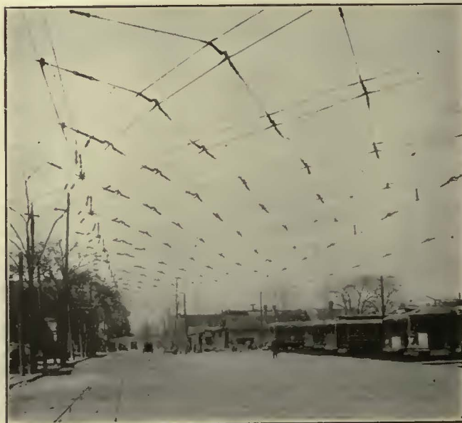
Overhead Connecting Curve Construction at Butler Street Carhouse in Atlanta
