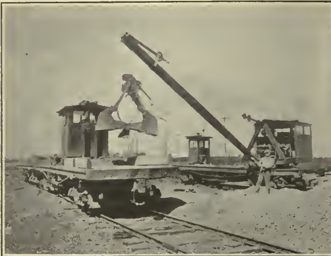
The Clamshell Is Used with the Long Boom
