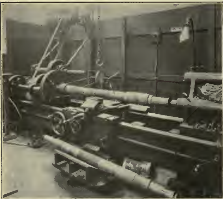
At Left, Belting Attachment to Old Lathe for Rotating Axle During Welding. At Right, Arrangement for Rotating Wheels for Building Up Flanges by Welding
