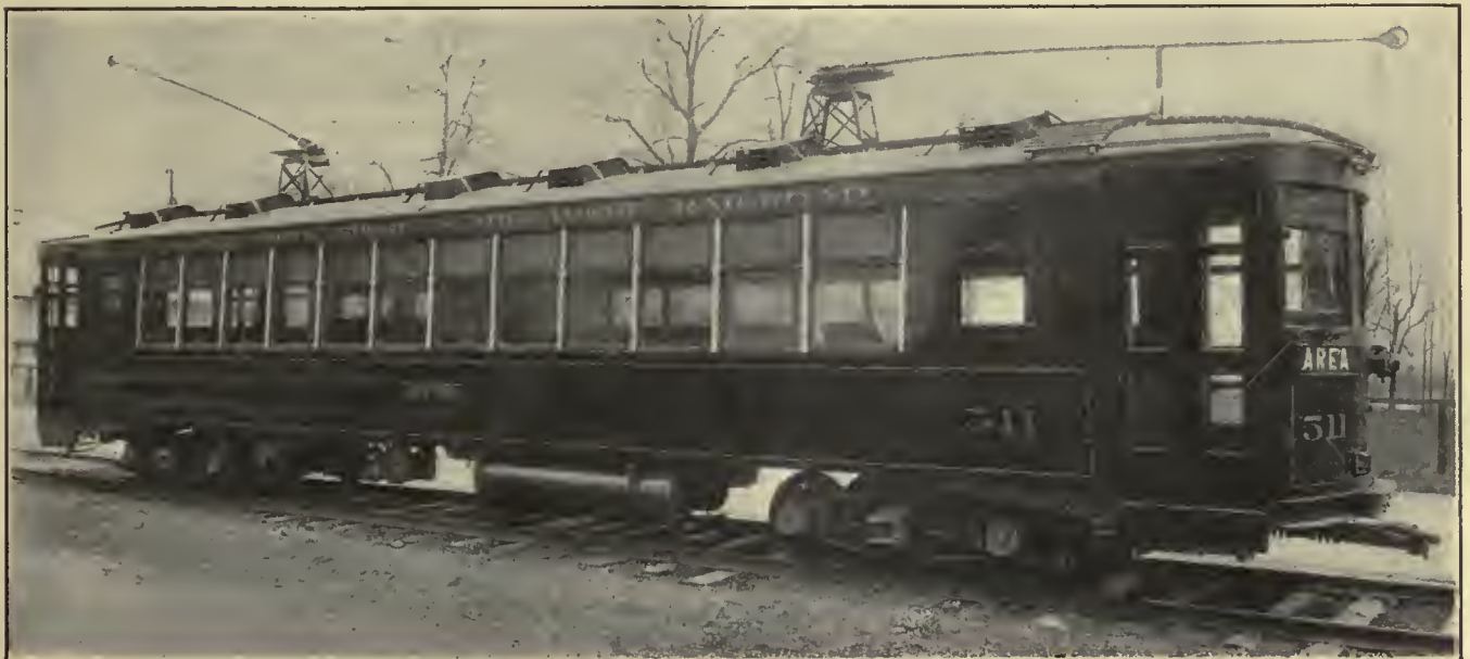
40,000-Lb., 47-Ft., Fifty-two-Passenger Car for Branch Line Service
