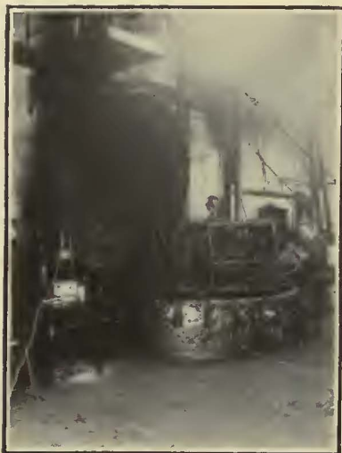
Impregnating Tank for treatment of Field Coils
