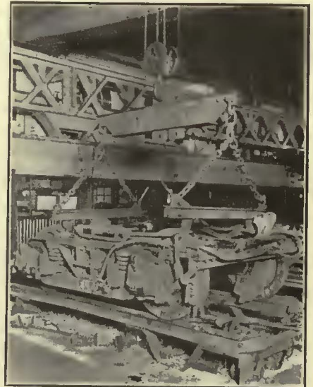
Rigging Used for Lifting Trucks by the Wheels
