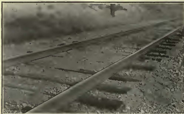
These Poles and Ties Treated with Wood Preservative Have Given Good Service At left, part of 2,500 creosoted poles set in 1907. In center, track on C. L. S. & S. B. Ry. with creosoted ties fifteen years old. At right, fifteen-year-old pole which is good for another fifteen years
