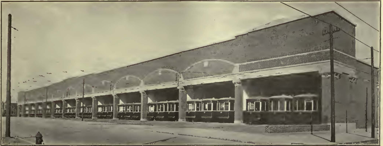
An Example of Recent Closed Storage Construction. Callowhill Carhouse, Philadelphia
