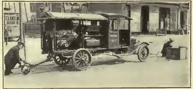
Welding and Grinding Operations Performed at the Same Time
