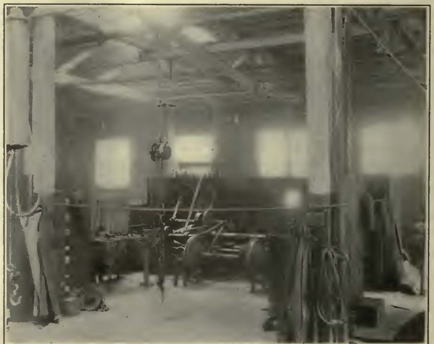
Welding Room in Shop of Lehigh Valley Transit Company
