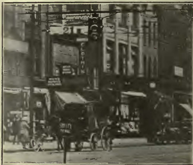
One of Eight Interlocked Signals at Successive Crossings
