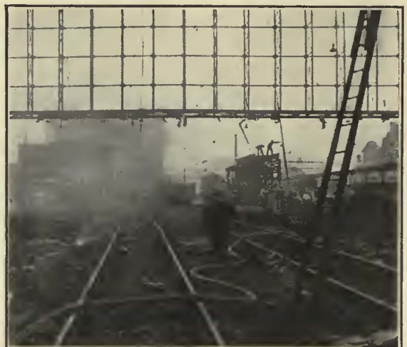
Crew of Tower Car Repairing Overhead Wires
