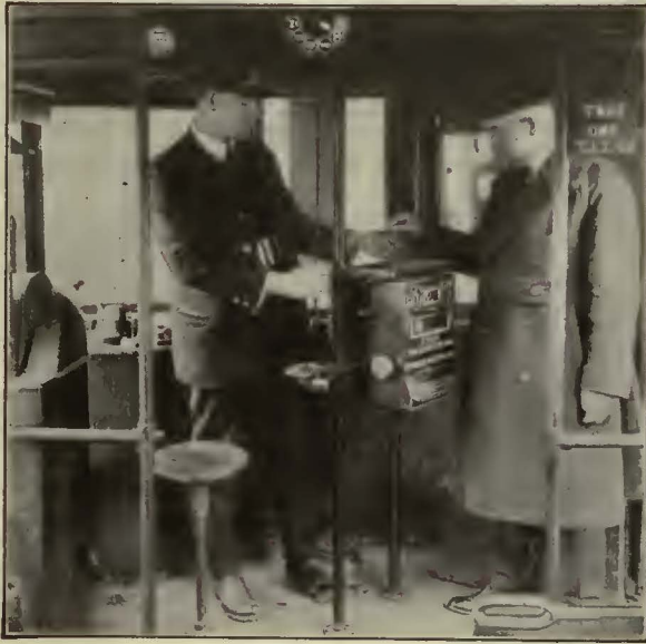
An Ohmer One Man Car Installation
