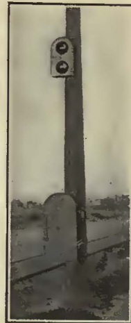
The Lenses Are Separate from the Operating Mechanism in This Signal
