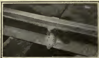
Feralite Welded Joint
