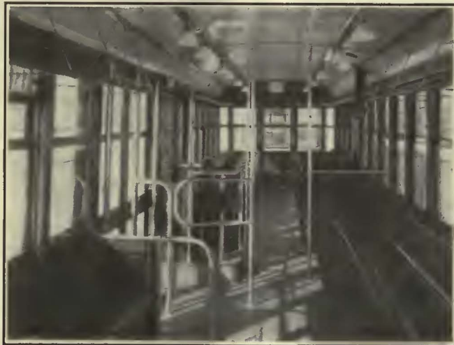
Center Well, Stanchions and Swinging Barrier, Grab Rail Over Longitudinal Seats, and Slat Seats
