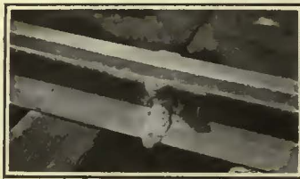
Feralite Welded Joint
