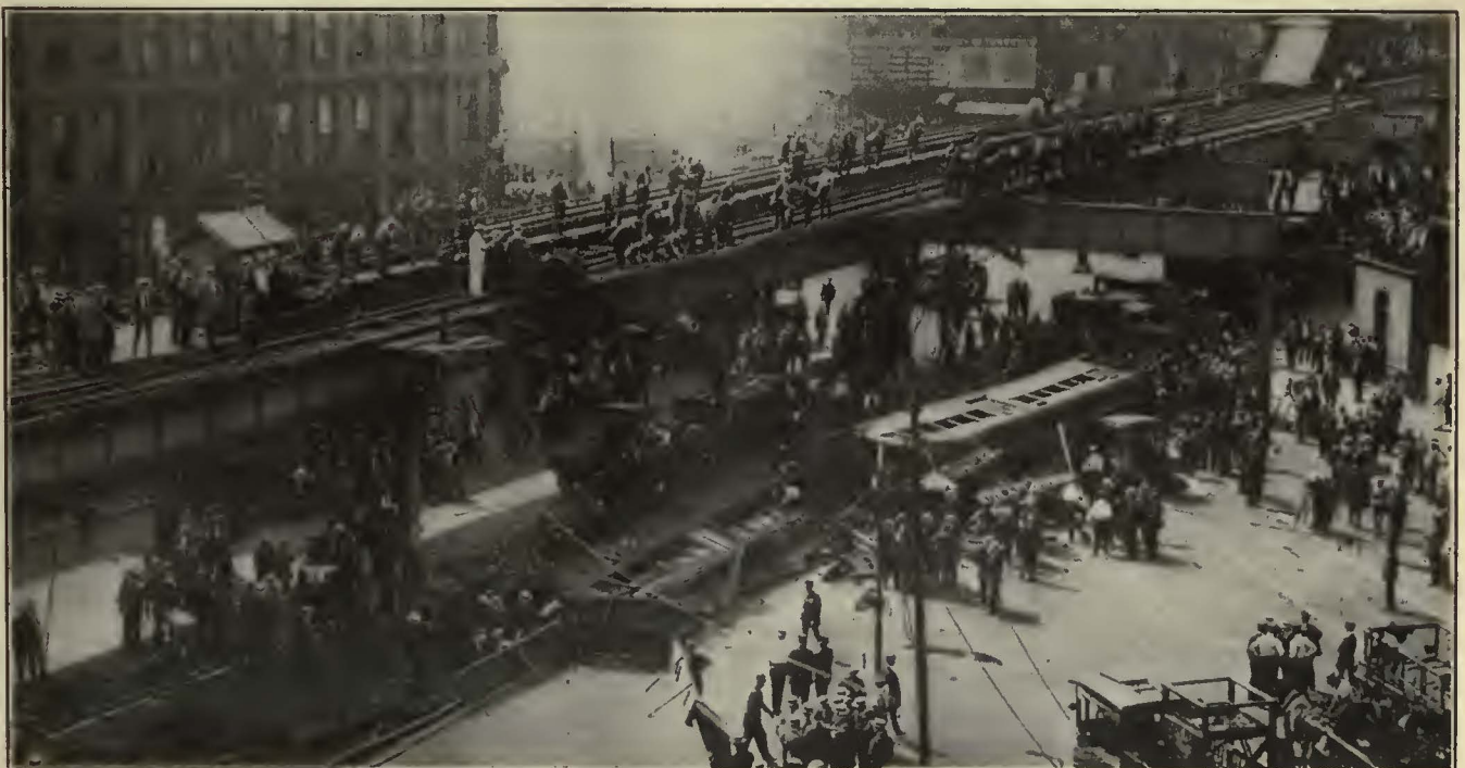
View Taken Shortly After Brooklyn Accident, Showing Officials Examining Elevated Structure Near Switch
