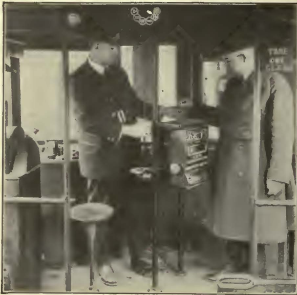
An Ohmer One Man Car Installation
