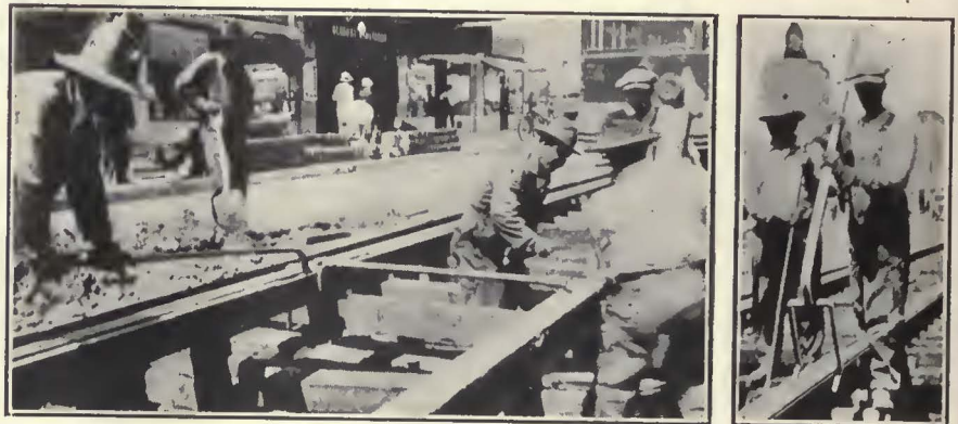
At Left, Holding a Tie in Position for Spiking. At Right, Form of Tie Bar Used by Pacific Electric Railway
