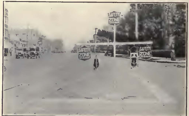
This Safety Zone Post Has Crossarms for Carrying Warning Notices and Lanterns
