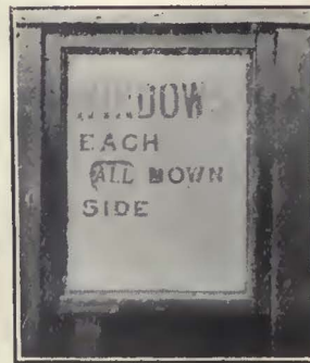
Sign in Window of Inspector's Shanty Gives Instructions as to Windows
