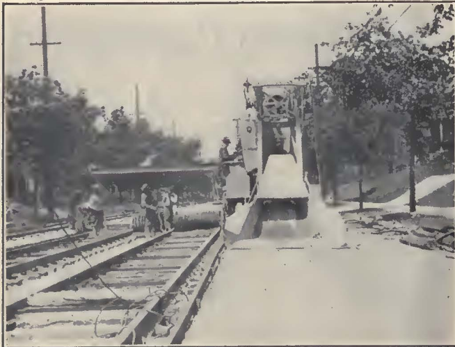
Left—Concrete Mixer in Working Position Ready to Receive Charge. Right—Special Forms Used Where Granite Header Blocks Are Employed for Flangeways
