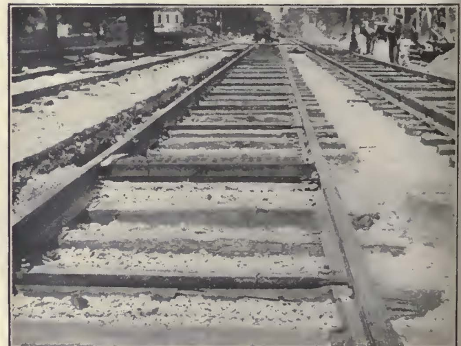
Left—Wire Mesh Reinforcing Placed 2\frac{1}{2} In. Below Finished Surface. Right—Track Construction; Note Wood Ties, Tie Rods, Rock Ballast and Track Drain. A Temporary Track Is Laid at One Side to Carry Traffic Past the Construction Work
