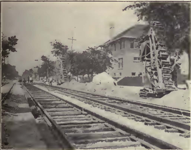
Left—Material Distribution and Equipment Arrangement for Concrete Paving Work in Milwaukee. In the Foreground Is the Crushed Stone and Loader; Beyond the Cement Is Piled; then the Sand and Sand Loader, and in the Background the Concrete Mixer. Right—Truck Tractor Receiving Measure of Gravel at Loader
