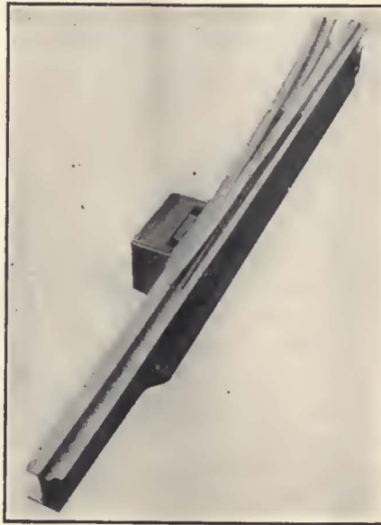
The Moving Part of This Switch Consists of Two Tongues and a Camshaft
