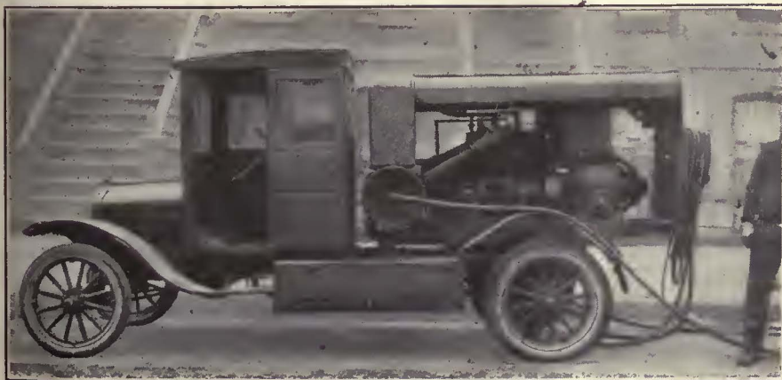
Air Compressor for Trackwork Mounted on Truck
