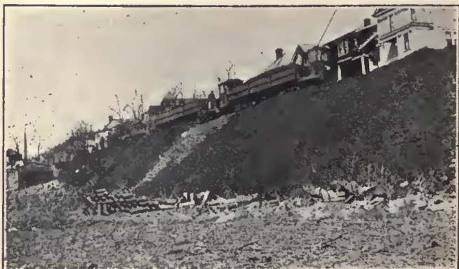
Filling in a Deep Ravine with the Ashes
