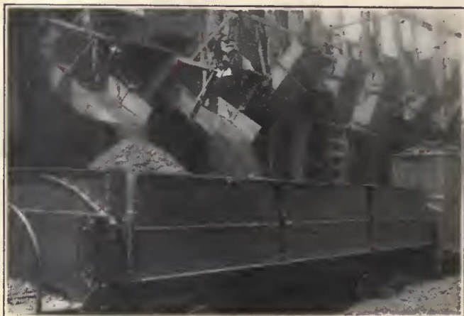
Loading Ashes at the Power House Hoppers
