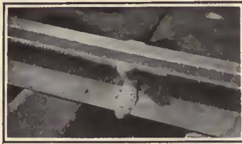
Feralite Welded Joint
