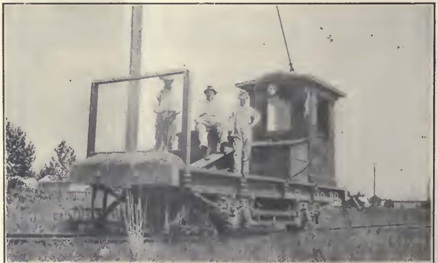
Steel Cable Sections Fastened to a Rotating Shaft Cut Weeds from Between the Rails
