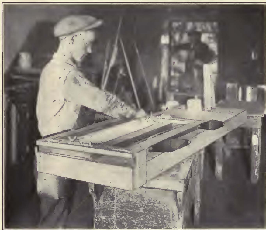
Squeegeeing White Lead Through Silk Screen Stencil in Sign Lettering Work
