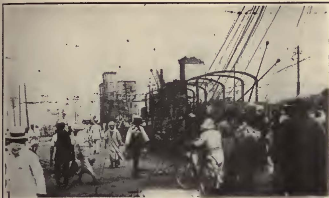
No. 1. Many Cars Were Completely Burned in the Fire Following the Tokio Earthquake
