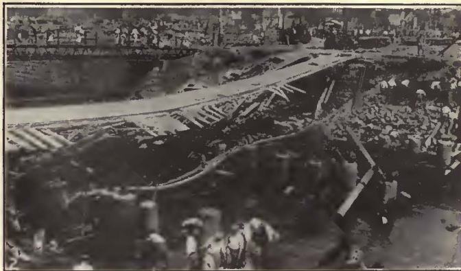
No. 2. A Number of Bridges Collapsed Completely. The Men in the Foreground Are Military Engineers
