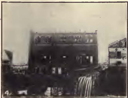
No. 4. The Yuraku Street Substation Was Completely Guttled by Fire. This Is One of the Tokio Stations Lost
