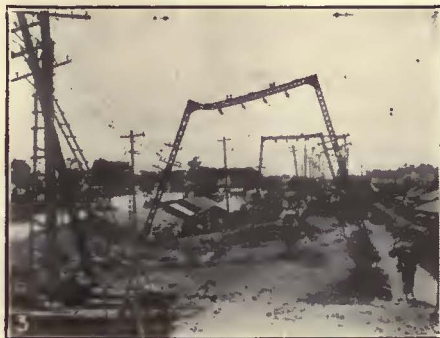
No. 3. The Line of the Keihin Electric Railway Was Destroyed by the Earthquake
