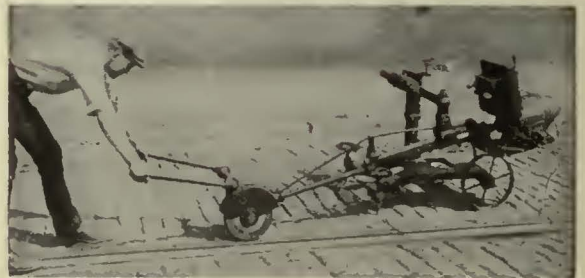
“Hercules” Rail Grinder
