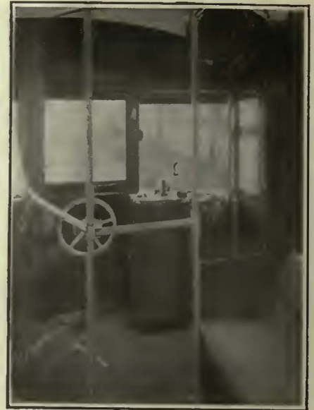
Motorman Located Right-Hand Corner of Leading Car. Brake Valve Piping Inclosed in Dash to Give More Knee Room
