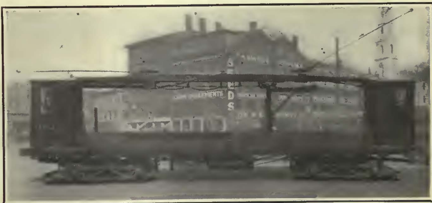
A Compressed Air Hoist Suspended from the Center Beam Does the Lifting Work of This Derrick Car
