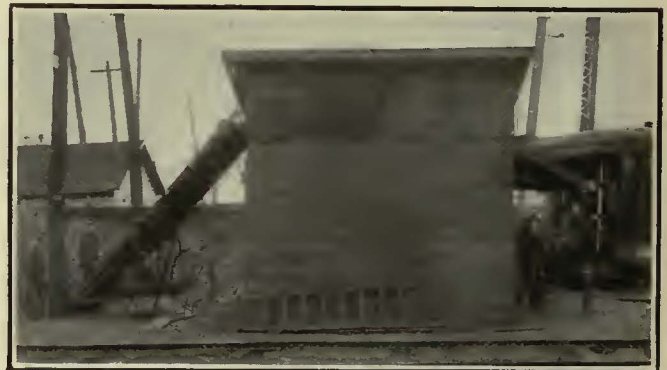
Coal-Handling Equipment for Supplying Car Heaters
