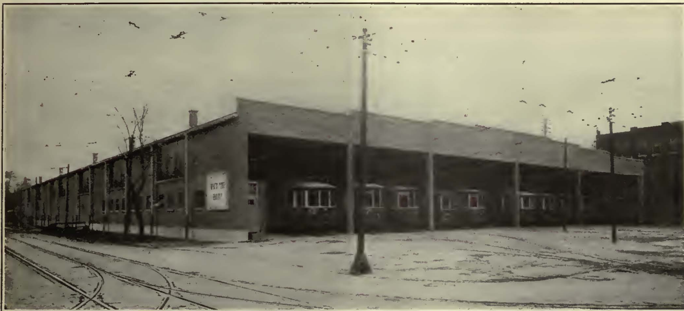
Louisville Carhouse from the Corner of Fourth and Avery Streets. A Reinforced Concrete Roof Is Placed Over the Entire Carhouse, but End Doors Are Not Provided
