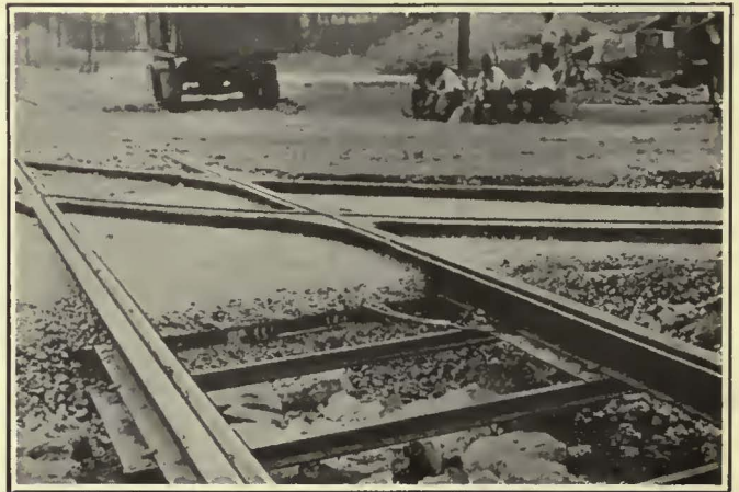
At Left—For Hand-Finished Paving Such as This a Greater Slump Is Permissible. At Right—A Moderately Dry Mixture of 1:2½:5 Concrete on Harrisburg, Pa., Track
