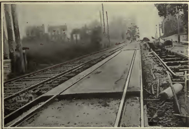
At Left—For Hand-Finished Paving Such as This a Greater Slump Is Permissible. At Right—A Moderately Dry Mixture of 1:2½:5 Concrete on Harrisburg, Pa., Track
