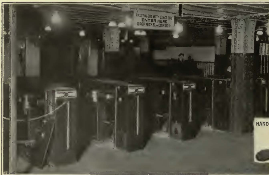
Latest type Perey Automatic fare collecting and registering passimeters used by Brooklyn-Manhattan Transit Corp.
