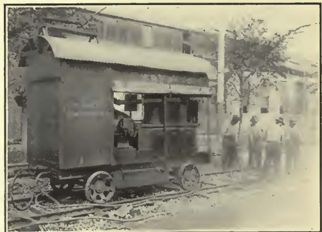
Heavy-Duty, Slow-Speed Air Compressors Are Used for Field Work
