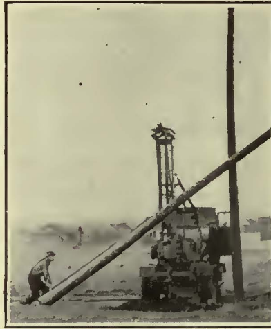
At Left, Digging a Hole. Each Load of Dirt Brought Up by the Auger Is Thrown to One Side. In Center, One Man Guides the Pole as It Is Raised. At Right, After the Pole Is Raised It Is Set in Position by the Machine
