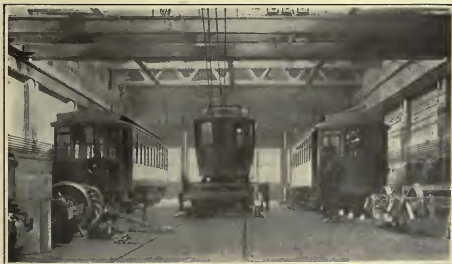
All Heavy Equipment Is Handled by a 10-Ton Crane
