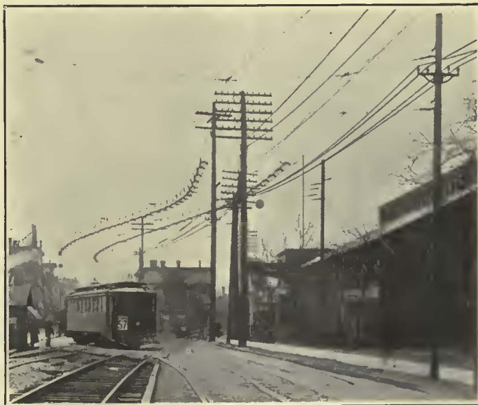
Left—Concrete Pole Installation at Charleroi, Pa., Pittsburgh Railways. Center—A Particularly Helpful Installation of National Trolley Guard on a Reverse Curve Crossing with the B. & O. R.R. on Second Avenue, Pittsburgh. Right—Typical Automatic Signal Installation of the Pittsburgh Railways. This Particular Installation is on the Beachview Route
