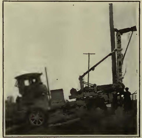
At Left, Digging a Hole. Each Load of Dirt Brought Up by the Auger Is Thrown to One Side. In Center, One Man Guides the Pole as It Is Raised. At Right, After the Pole Is Raised It Is Set in Position by the Machine
