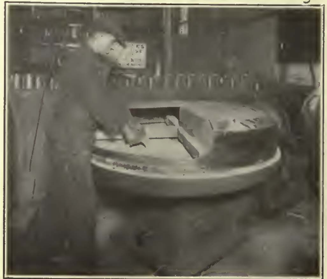
Finishing Axle Bearing Shells by Use of a Surface Grinder Multiplies Production by Four
