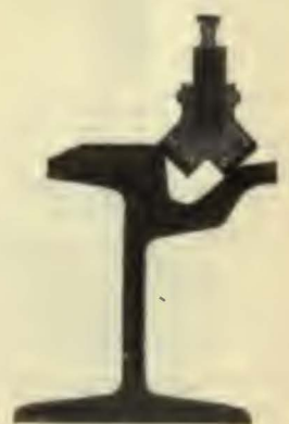
Bar in Place on "Girder" Rail Showing Saw Blade Contact
