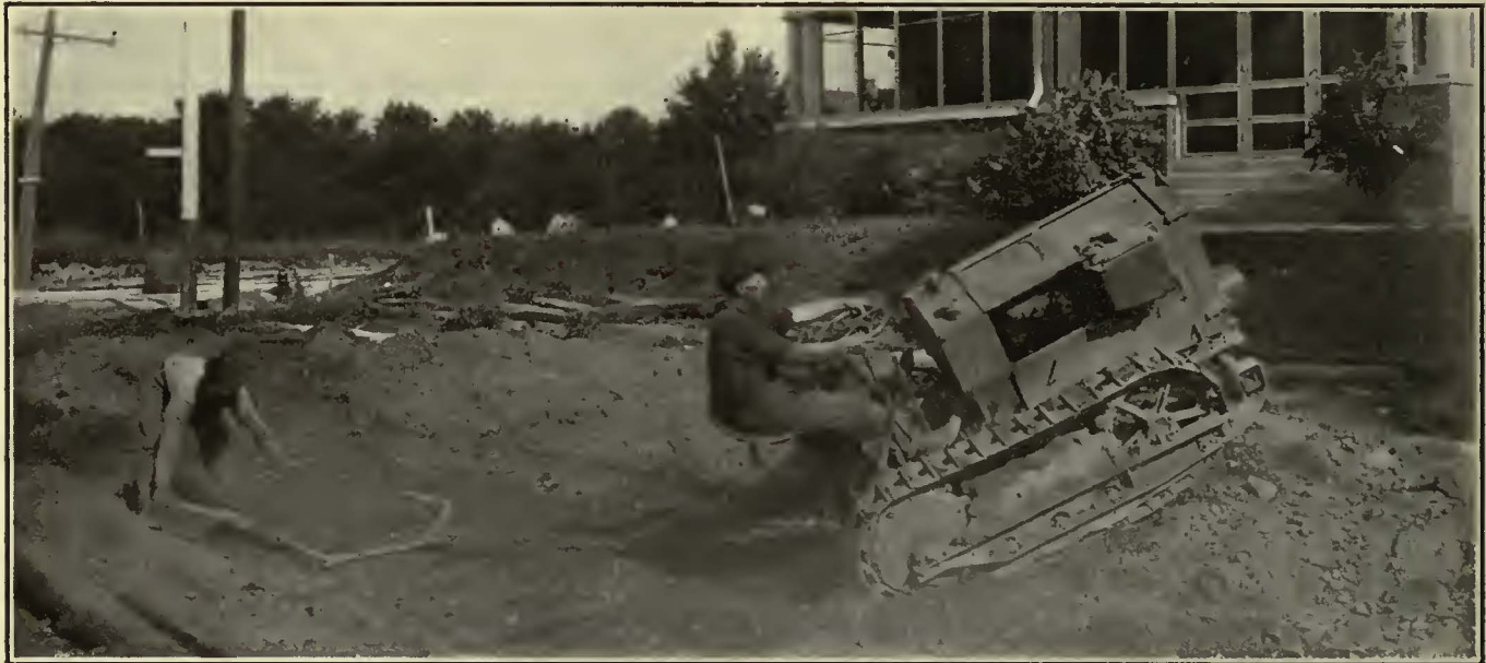
The Tractor Speeds Up Grading and It Will Go Anywhere
