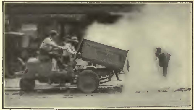
Holst Dump Tractors Are Particularly Useful in Distributing Paving Material
