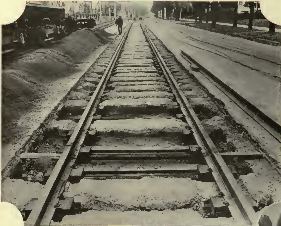
Recent Installations of Dayton. Resilient Tracks
