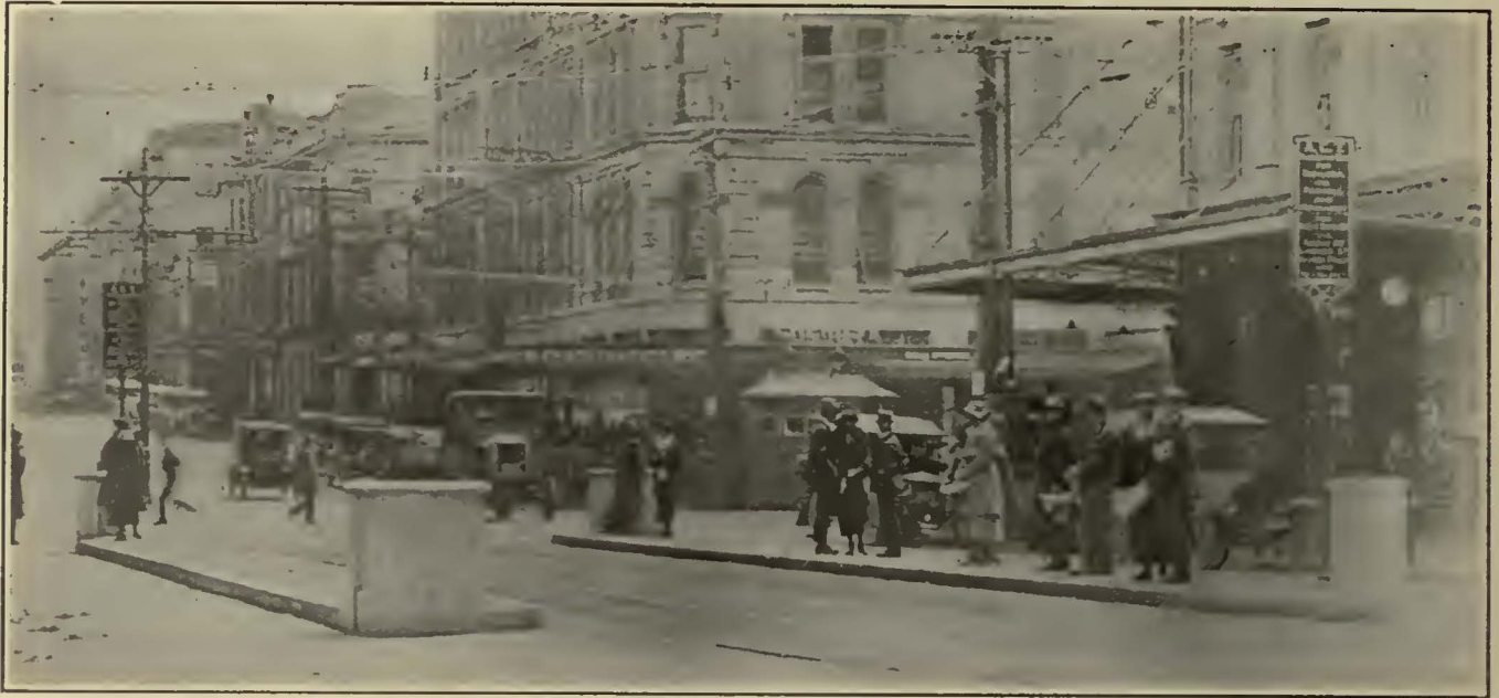
Substantial Waiting Platforms of Concrete Are a Feature of Some of the Downtown Streets in Auckland
