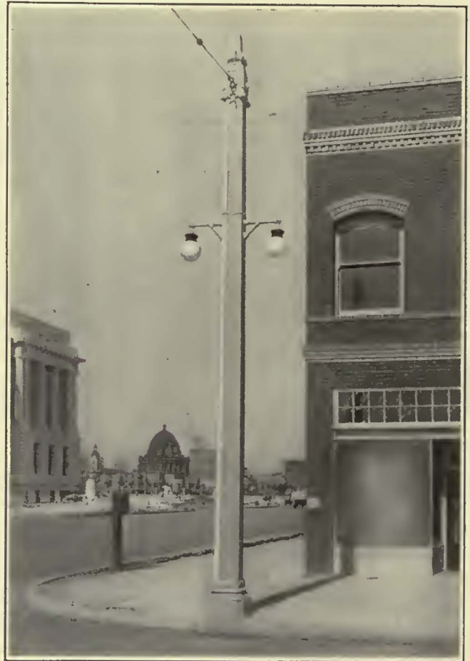
Type of Concrete Pole Used by Municipal Railway of San Francisco
