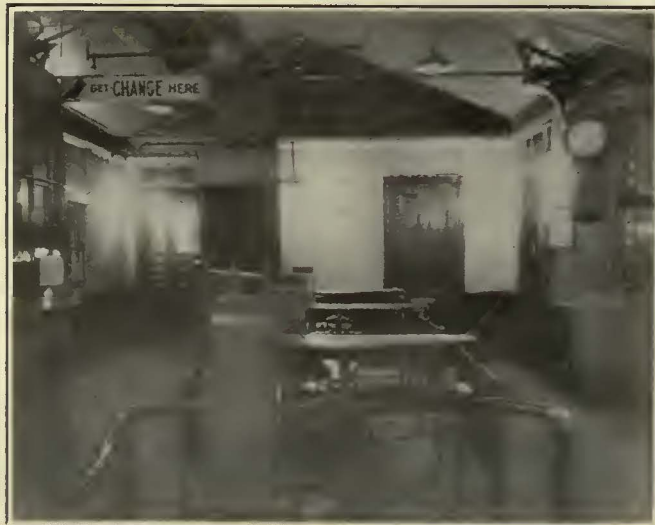
Old and New Method of "L" Station Lighting Ten 40-watt lamps on wall brackets (left) have been replaced with four 75-watt ceiling lamps with reflectors (right), giving 350 per cent better illumination over the turnstiles, without glare.
