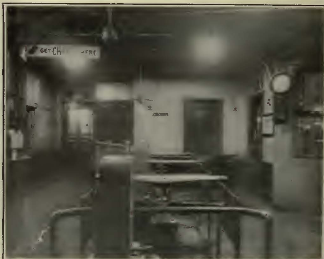
Old and New Method of "L" Station Lighting Ten 40-watt lamps on wall brackets (left) have been replaced with four 75-watt ceiling lamps with reflectors (right), giving 350 per cent better illumination over the turnstiles, without glare.
