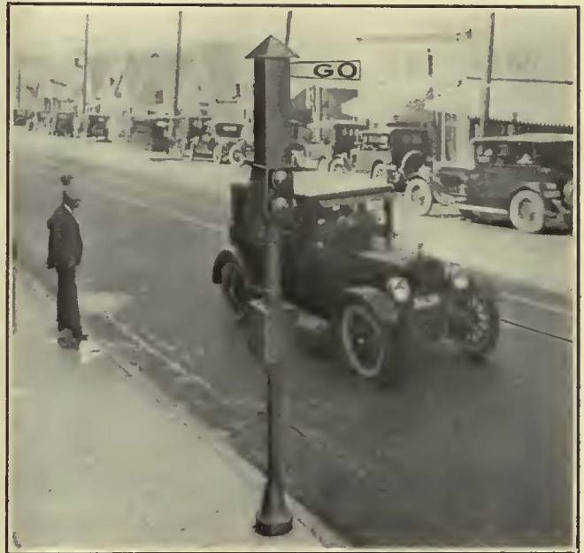
A Signal Standard of This Type Is Used at Each of the Four Corners of Every Street Intersection in the Congested District of Los Angeles
