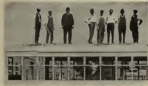
The weight of eight men is easily supported by the HASKELITE roof panels. Yet this material weighs 30% less than tongue and groove poplar roofing.
