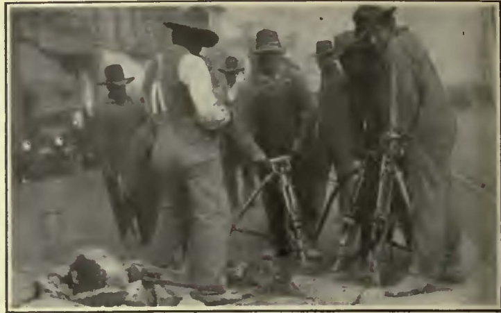
Cutting Up a 9-In. Solid Concrete Pavement with the Pneumatic Cutters
