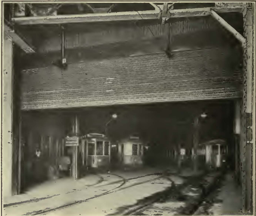
Through the Installation of This Rolling Door at the Carhouse Entrance a Considerable Saving of Coal Has Been Effectuated
