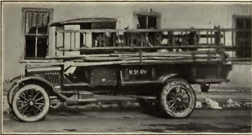
When Making Repairs to the Overhead Lines the Ladder Is Taken Off the Hooks of the Nushua Line Truck and Fastened in a Vertical Position
