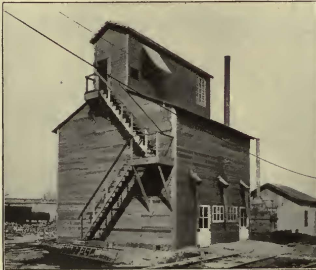
This illustration above shows a completed 200-ton capacity sand dryer and storage house—"sand house"—for short. We furnished the dryer, feed elevator, hot sand elevator, rotary screen with hopper, distributing pipes from hopper, discharge gates and pipes and structural steel frame. The Street Railway Co. provided the foundations and lumber.
