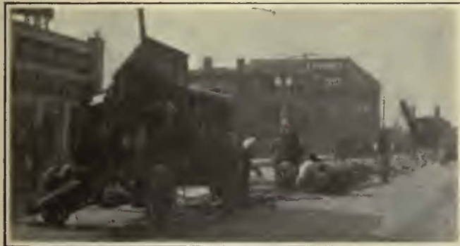
Steam Shovel Loading Broken Pavement When a Second Track Was Being Laid on Sixth Street
