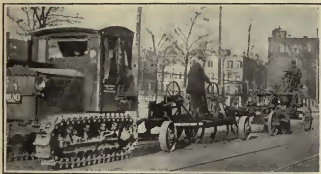
The Projecting Teeth Break Up High Ice Between the Rails
