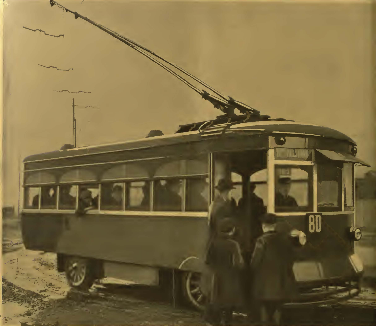
Brill trolley bus with GE-258 Motors and foot-operated M control.
