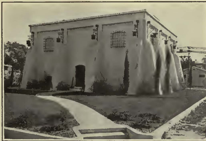
These Designs of Noiseless Substations of the Los Angeles Railway Show the Architectural Treatment. Top, Left—West Adams. Top, Right—Melrose. Bottom—Garvanza
