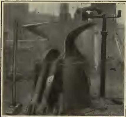
Turnbuckle in Position for Closing in Ends
