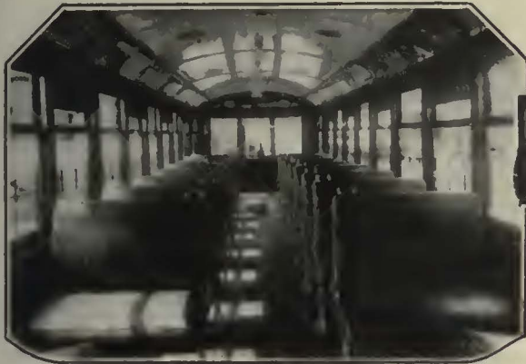
Youngstown and Suburban Railway operated by Day & Zimmerman, Inc., use HASKELITE roofs and PLYMETL sides without head linings or side linings. Cars built by G. C. Kuhlman Car Company.
