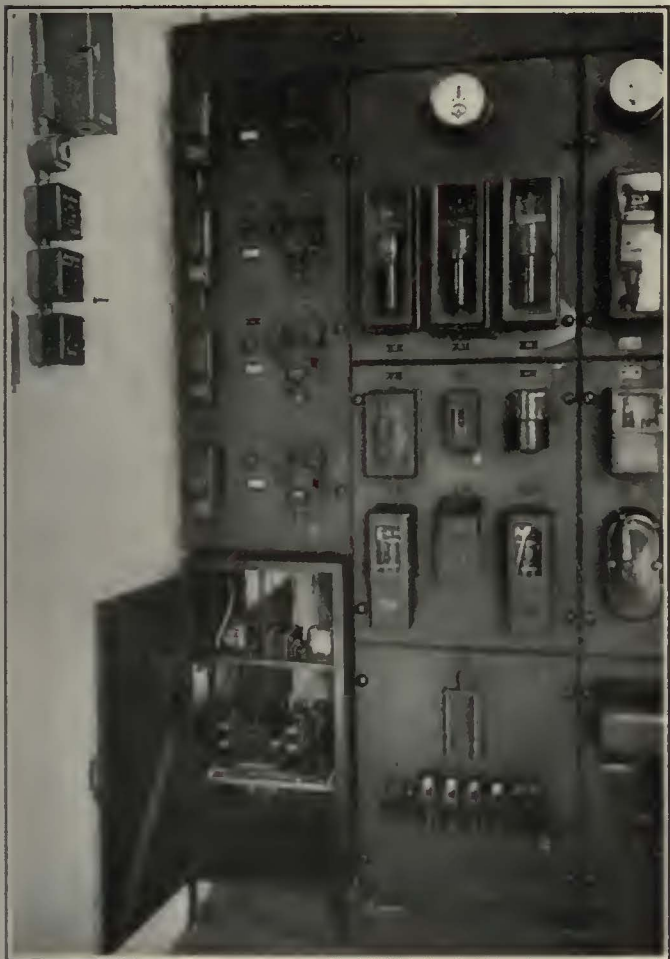
Above, Full Supervisory Control Apparatus Is Carried on the Left-Hand Panel of the Switchboard. The 2,000-Kw. Converter Is Shown in the Foreground
