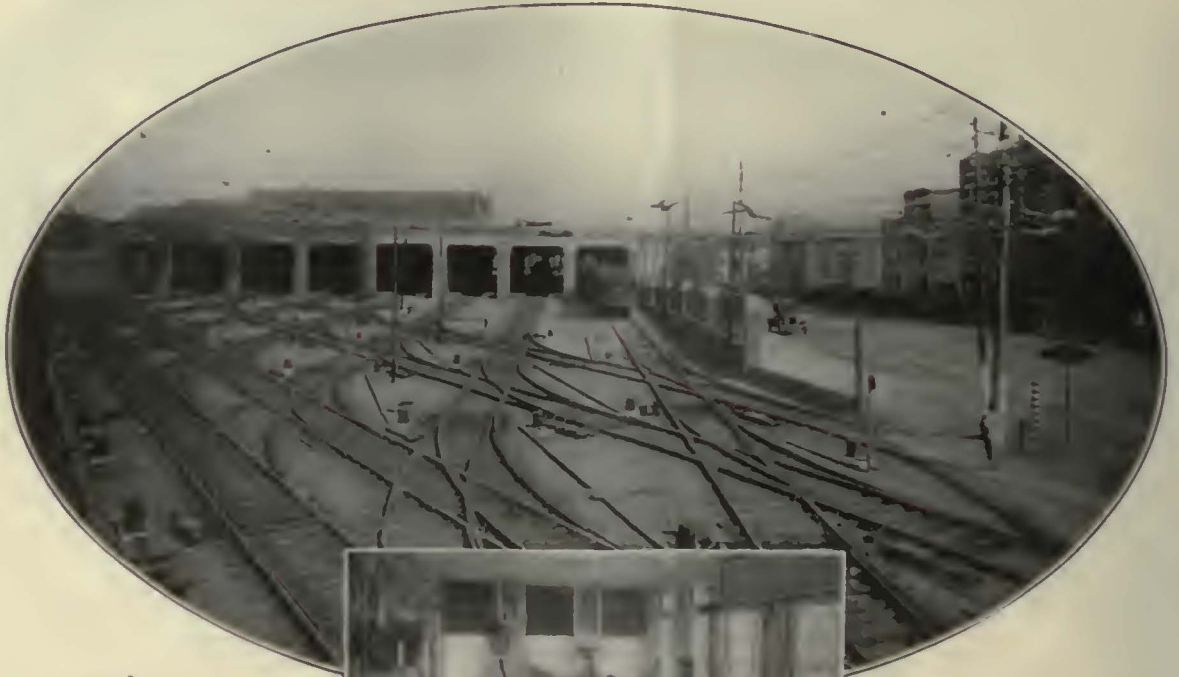
Electro-Pneumatic Interlocking at Terminal Station of Philadelphia & West Chester Traction Co.
