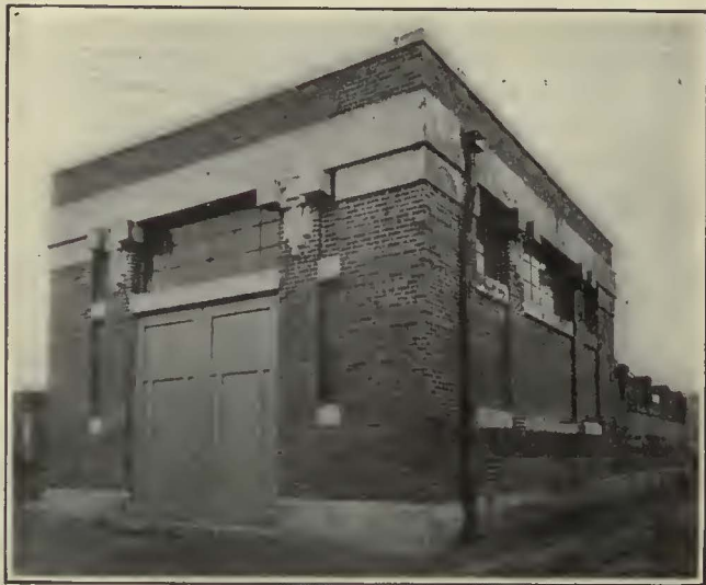
Central Street Automatic Substation of the Chicago Rapid Transit Company, in Which the Supervisory Equipment Is Installed
