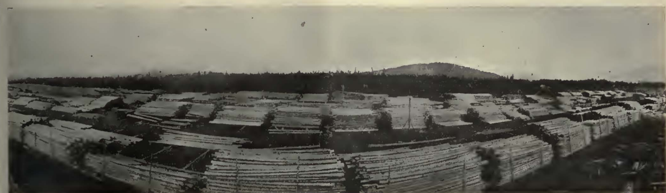
THE KOOTENAI, IDAHO, POLE YARD One of the five immense Weyerhaeuser storage yards where poles are seasoned and prepared for shipment.
