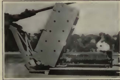
Resistor Installed on Roof of Car
