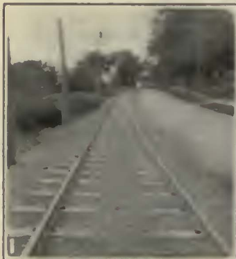
No. 1. Trial Installation of Concrete Ties on the Bangor Railway & Electric Company. No. 2. The Ties Are Made of Concrete Blocks Connected by Steel Rods. No. 3. The Special Spikes Used Are Made in Two Parts Held Together by a Cotter Pin
