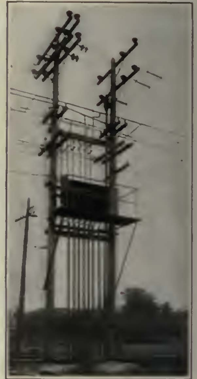
At Left, All High-Tension Apparatus Is Located in an Adjacent Outdoor Court, Enclosed by a Brick Wall and Wire Fence. At Right, Laterals and Switches Connect the Duct Line from the Substation with the Overhead at the Railway Right-of-Way
