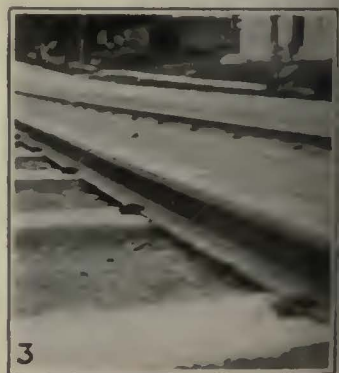
No. 1. Trial Installation of Concrete Ties on the Bangor Railway & Electric Company. No. 2. The Ties Are Made of Concrete Blocks Connected by Steel Rods. No. 3. The Special Spikes Used Are Made in Two Parts Held Together by a Cotter Pin
