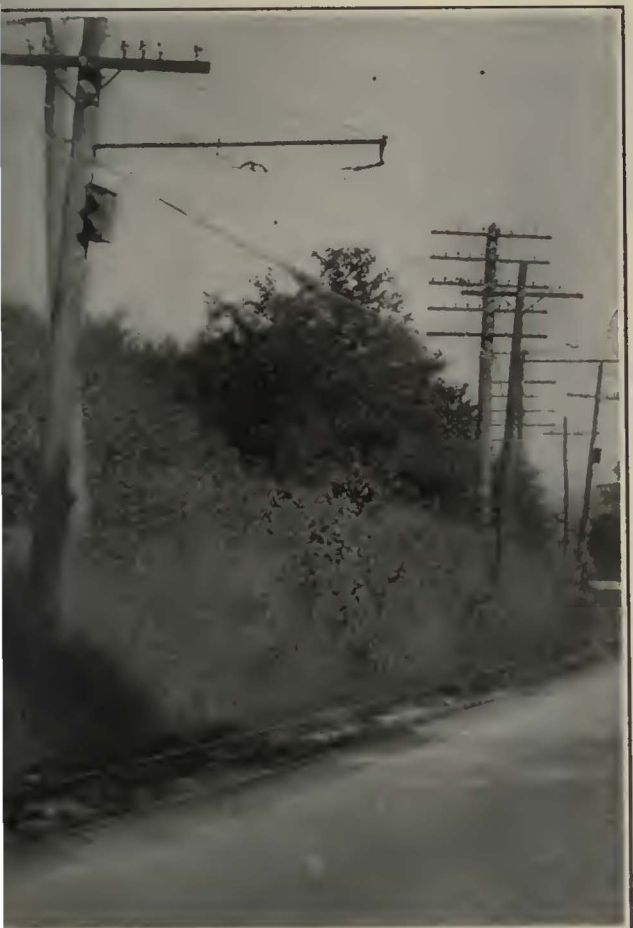
These Signals Duplicate Indications at Entrance to the Block
