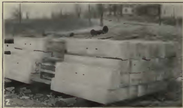
No. 1. Trial Installation of Concrete Ties on the Bangor Railway & Electric Company. No. 2. The Ties Are Made of Concrete Blocks Connected by Steel Rods. No. 3. The Special Spikes Used Are Made in Two Parts Held Together by a Cotter Pin
