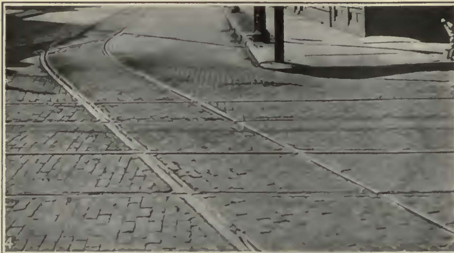
Examples of Thermit-Welded Special Work
