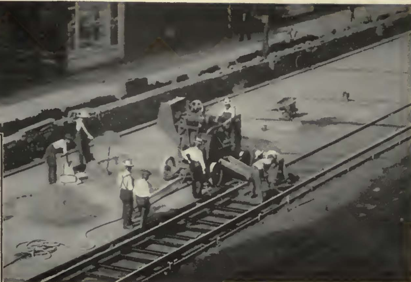
Main Street, Maitoon, Ills. Bituminous brick paving. Elastite Rail Filler both sides of car rails. City Engineer—John Goetz. Contractor—A. C. Loomis.
