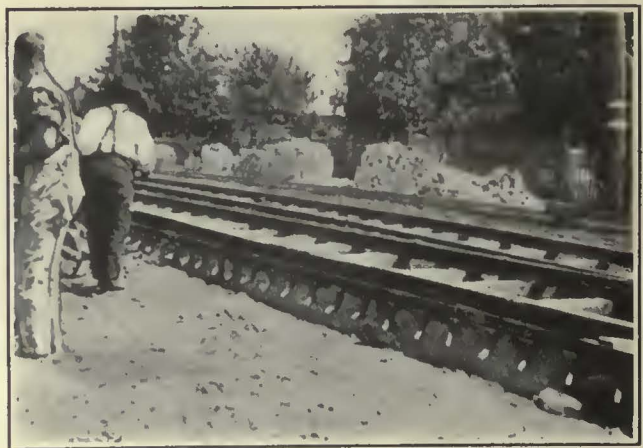
Showing How Godwin Steel Paving Guards Are Installed at Halifax
