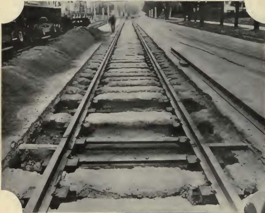
Recent Installations of Dayton Resilient Tracks
