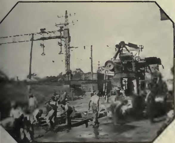
Spaces between and along trolley tracks on the Boston Post Road at Darien, Conn. Eighteen hours after pouring, the pavement was opened to traffic, including heavy commercial trucks. Had ordinary concrete been used, weeks would have been lost
