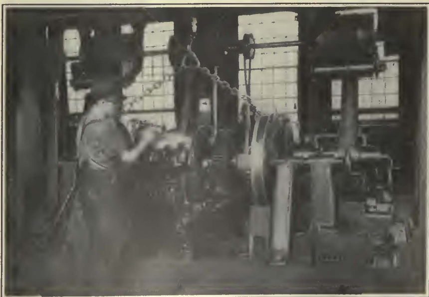
One Man Grinds 30 to 35 Pairs of Wheels per Day on This Norton Grinder in the Twin City Rapid Transit Company's Shop
