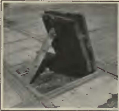
Section Raised, Showing How Lower Layer Is Hewn to Fit Bolt Heads, While Upper Layer Is Cut to Fit Head of Guard Rail
