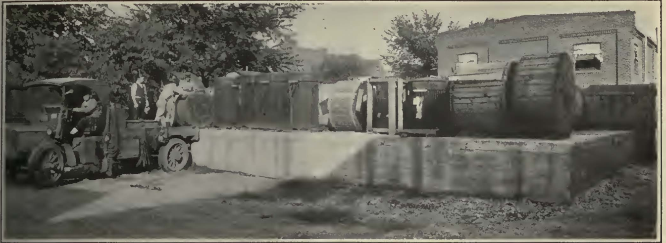
Concrete Platform for Storing Heavy Reels of Cable and Large Transformers. Two-Ton Reels and Large Transformers Can Be Easily and Quickly Loaded and Unloaded from This Platform
