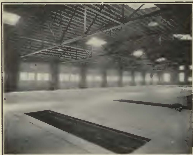
Interior of the Garage at Decatur, Showing the Inspection Pits
