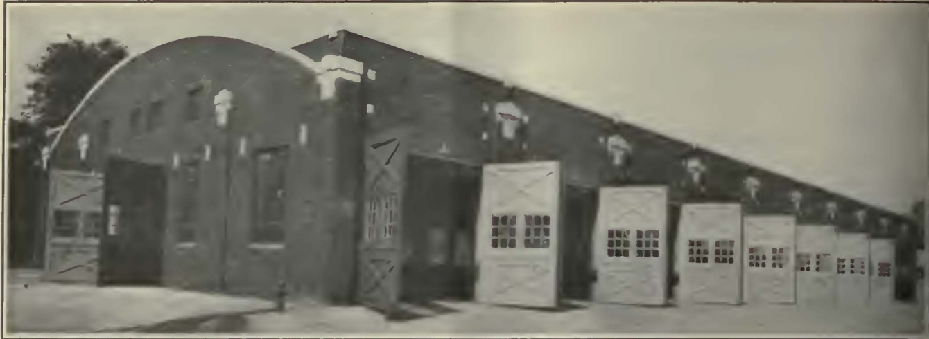
A Modern Garage with 16,000 Sq.Ft. of Floor Space Has Been Built to House the Buses
