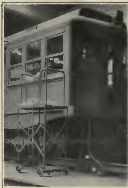
Easily Movable Carriage Which Has Doubled the Efficiency of the Exterior Car Cleaners
