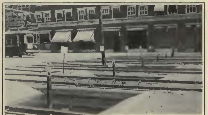
Arrangement of Pits and Red Lights to Prevent Unauthorized Entrance to Passenger Terminal from Street
