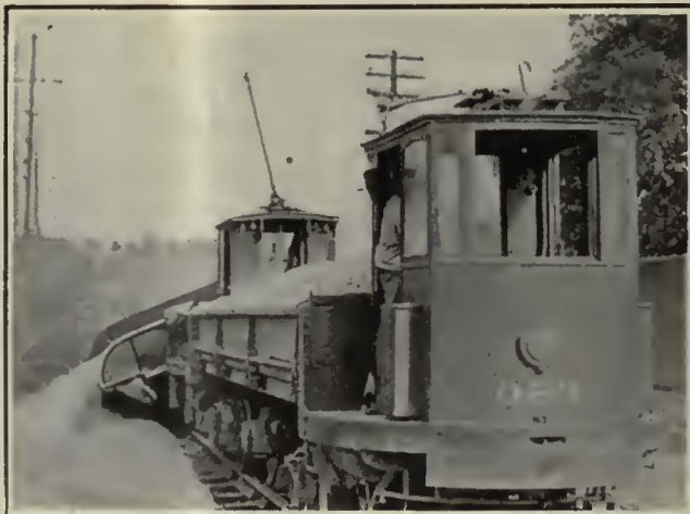
"Differential Two-Car Train. Trailer dumping load clear of trench."
