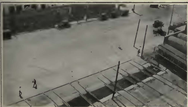
Arrangement of Pits and Red Lights to Prevent Unauthorized Entrance to Passenger Terminal from Street
