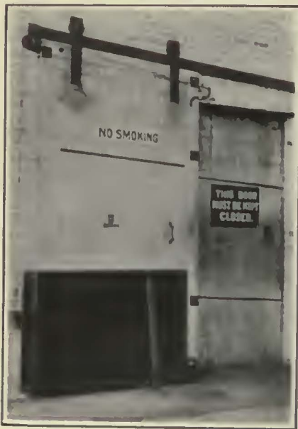
Sheet Steel, Reinforced Shield Protects the Fire Door from Materials and Equipment Which Might Render It Inoperative
