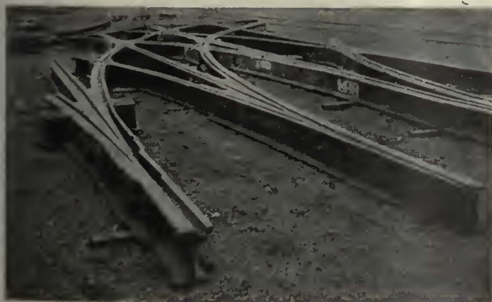
3-WAY SWITCH LAYOUT DESIGNED FOR AN EASTERN RAILWAY
