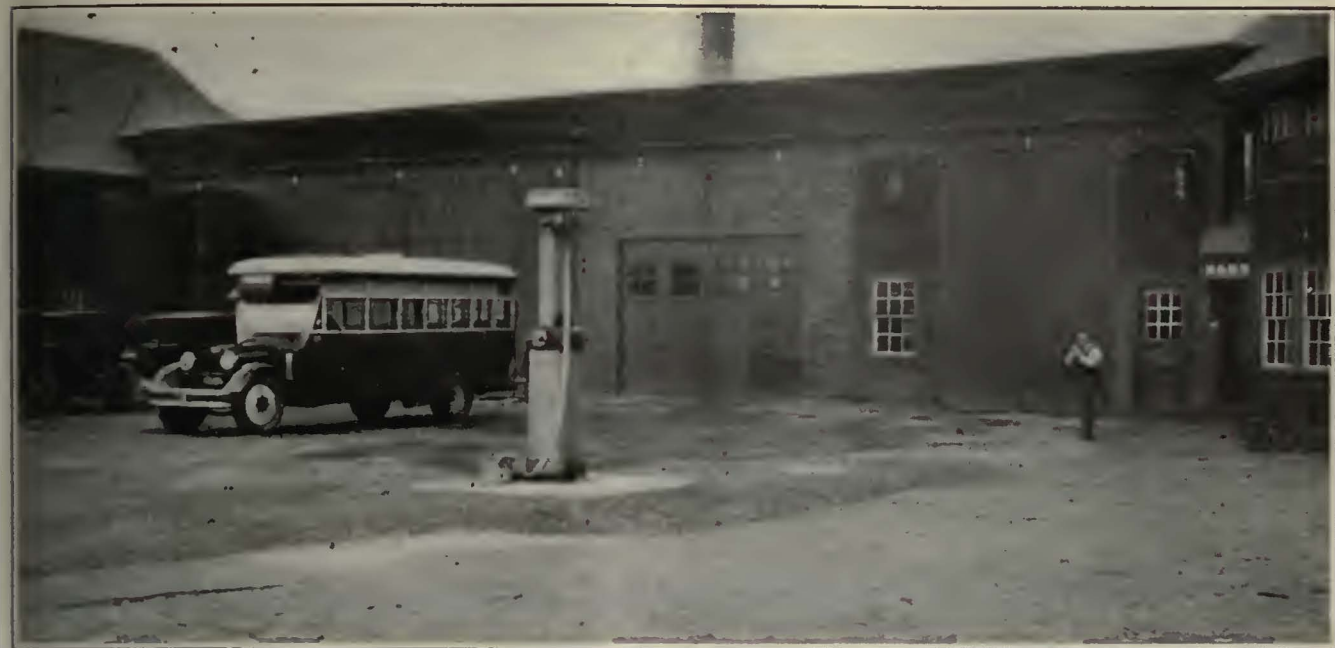
The North Lexington Carhouse Has Been Converted Into a Bus Garage
