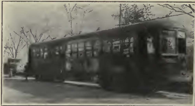
This 32-Ton Interurban Car Was Operated Over a New Concrete Roadbed 26 Hours After Its Construction
