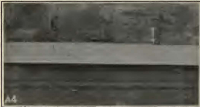
Bolted Joints Photographed in 1921 at Left and Again in 1924 at Right. In the Interval 535,000 28-Ton Cars Passed
