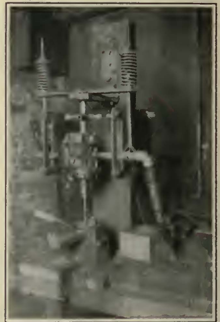
With This Supporting Arrangement a Pneumatic Drill Is Used for Drilling Small Parts on the Work Bench
