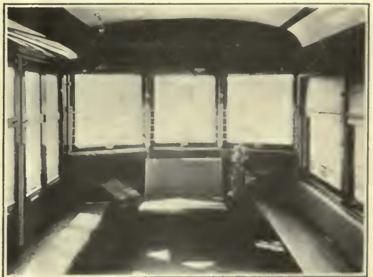
An Observation Section and a Baggage Compartment Are Provided in the I. T. S. One-Man Interurban Car
