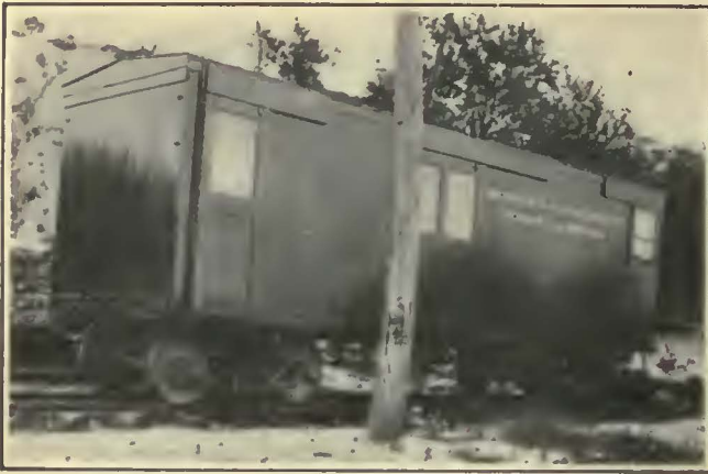
All of the Apparatus of This Portable Substation Has Been Placed Inside of the Car Body
