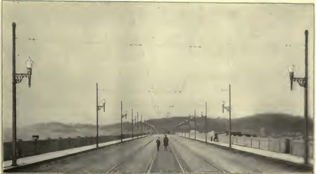
ELRECO Combination Railway and Lighting Poles on the Hopple Street Viaduct, Cincinnati, O. Over 27,000 ELRECO Poles are in use in this city
