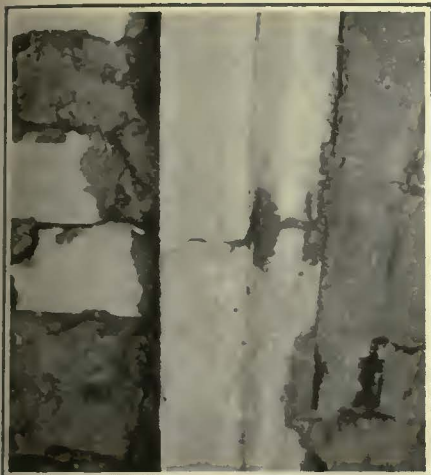
At Left, Cupped Rail Repaired by Adding New Material with an Arc Welder. At Right, Manganese Cross-Over Points, Built Up by Arc Welding. Such Repairs Have Stood Years of Service
