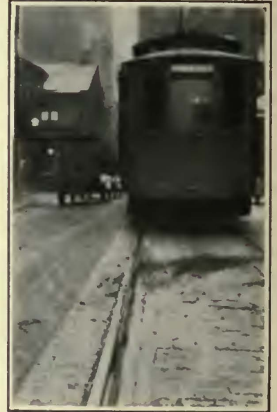
Appearance of Concrete Flangeway and Brick Pavement Used in Altoona
