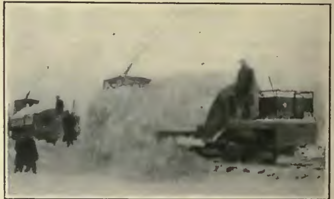
Dumping Snow at Manhole for Disposal After Removing It from the Streets of Toronto
